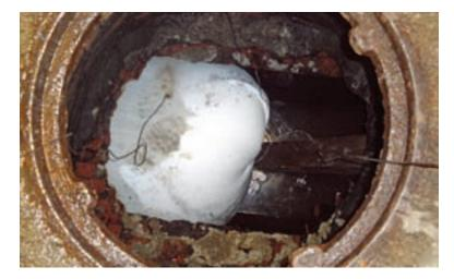
A wooden chock in the downstream manhole stops the liner's forward motion. A "soft end," or hold-back device, and hold-back rope control its rate of inversion and prevent an uncontrolled runaway. Right: The liner inverting down the pipe.
