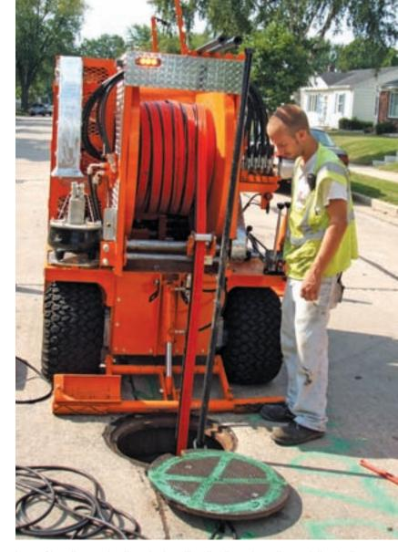
Lucas Bignell operates the winch pulling the liner down the mainline to the lateral where it will be installed.
