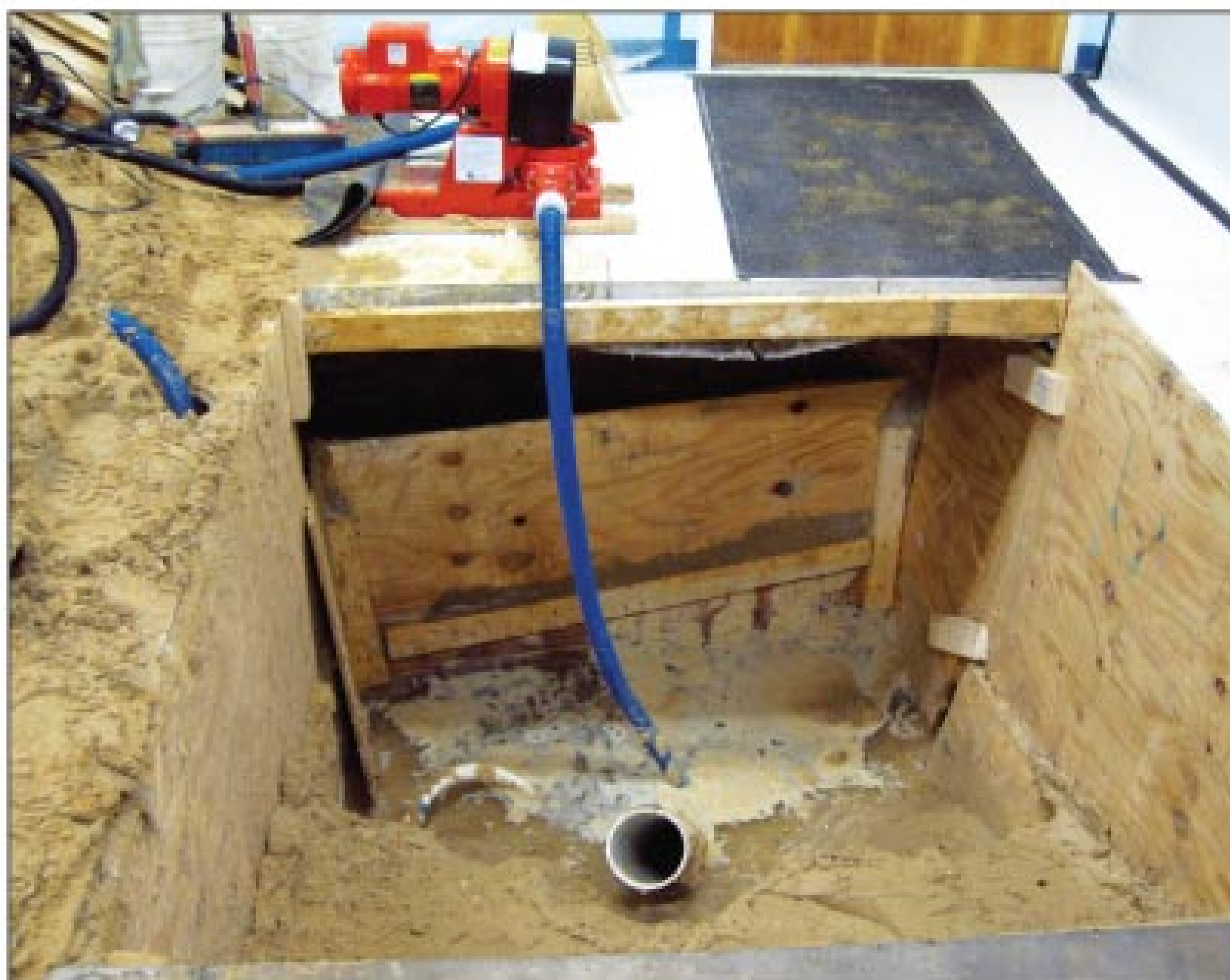
Tides influenced the water table in the 6-foot-square access pit in the nuclear medicine department.
