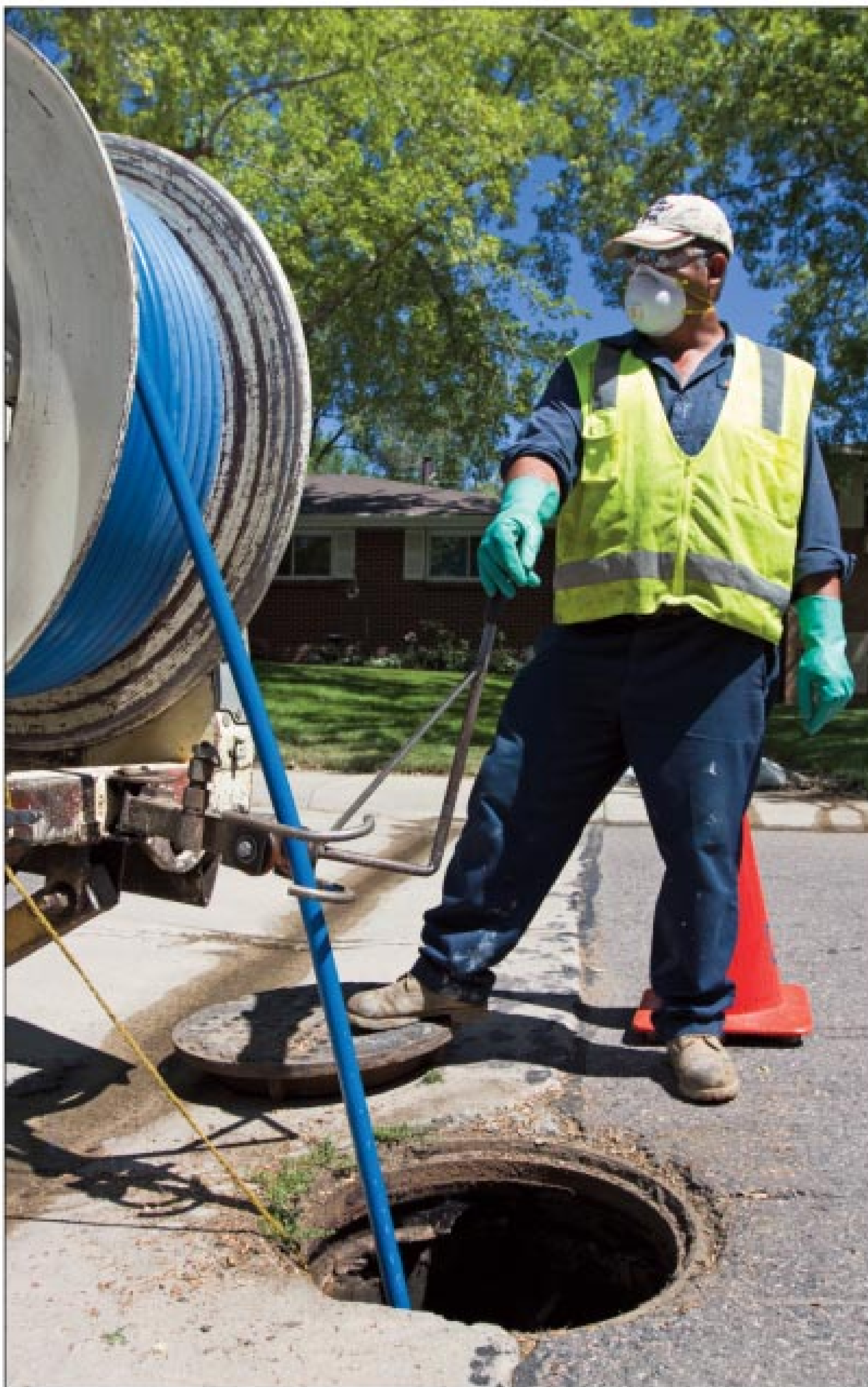
Upper photo: Everardo Canela pulls the hose slowly back to the truck, spreading the herbicide that will kill roots inside the pipeline. Lower photo: Inspection operator Leonard Josytewa watches video as foreman Mark Lei (not shown) lowers a chain cutter into a line.
