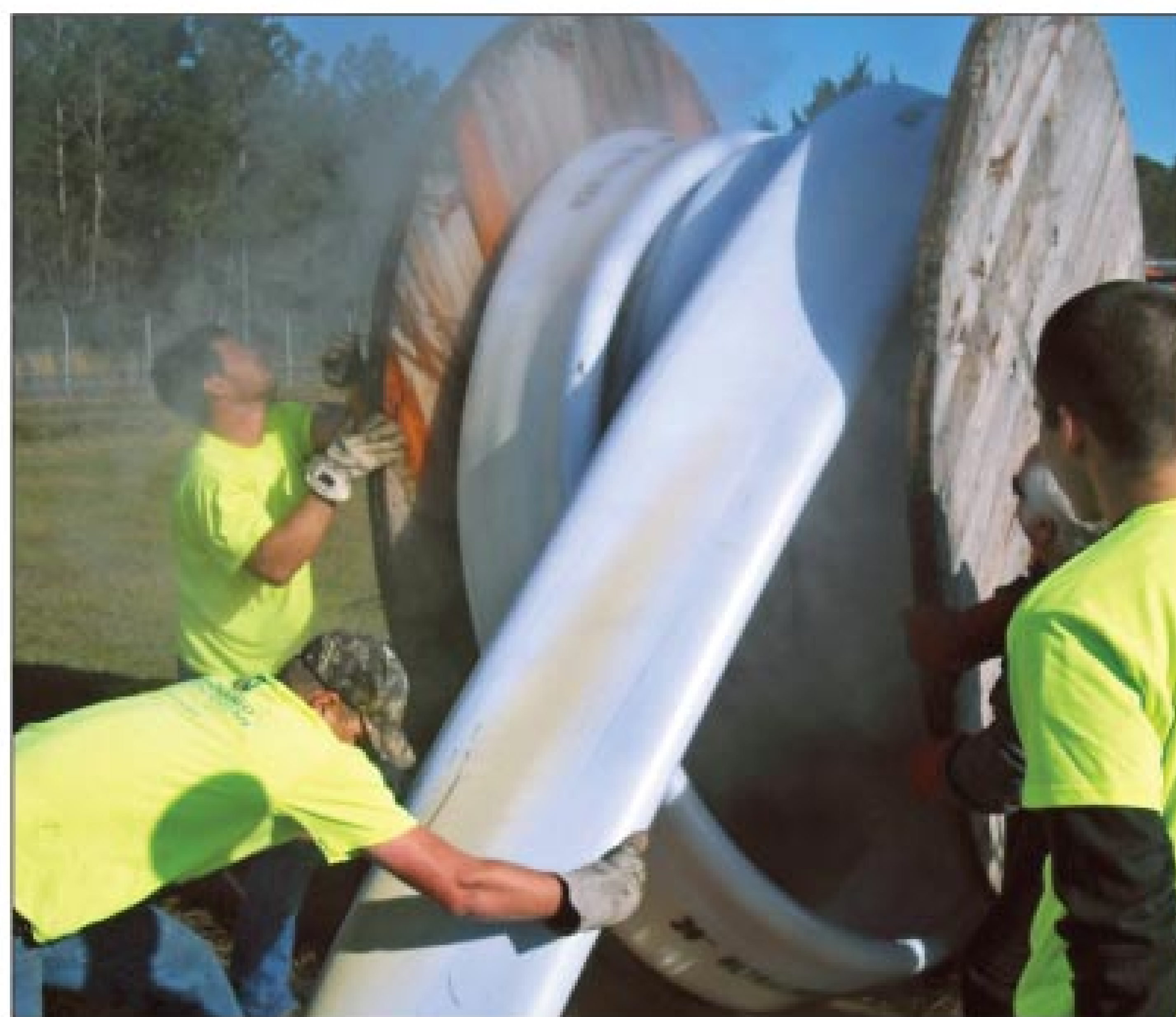
Top: The boiler truck generates steam that softens the SDR35 PVC alloy pipe, enabling it to be pulled off the spool and into the sewer. Below: Steam rises from the heated liner as workers from Engineered Lining Systems pull the head of the liner toward the manhole. (Photos courtesy of Engineered Lining Systems Inc.)
