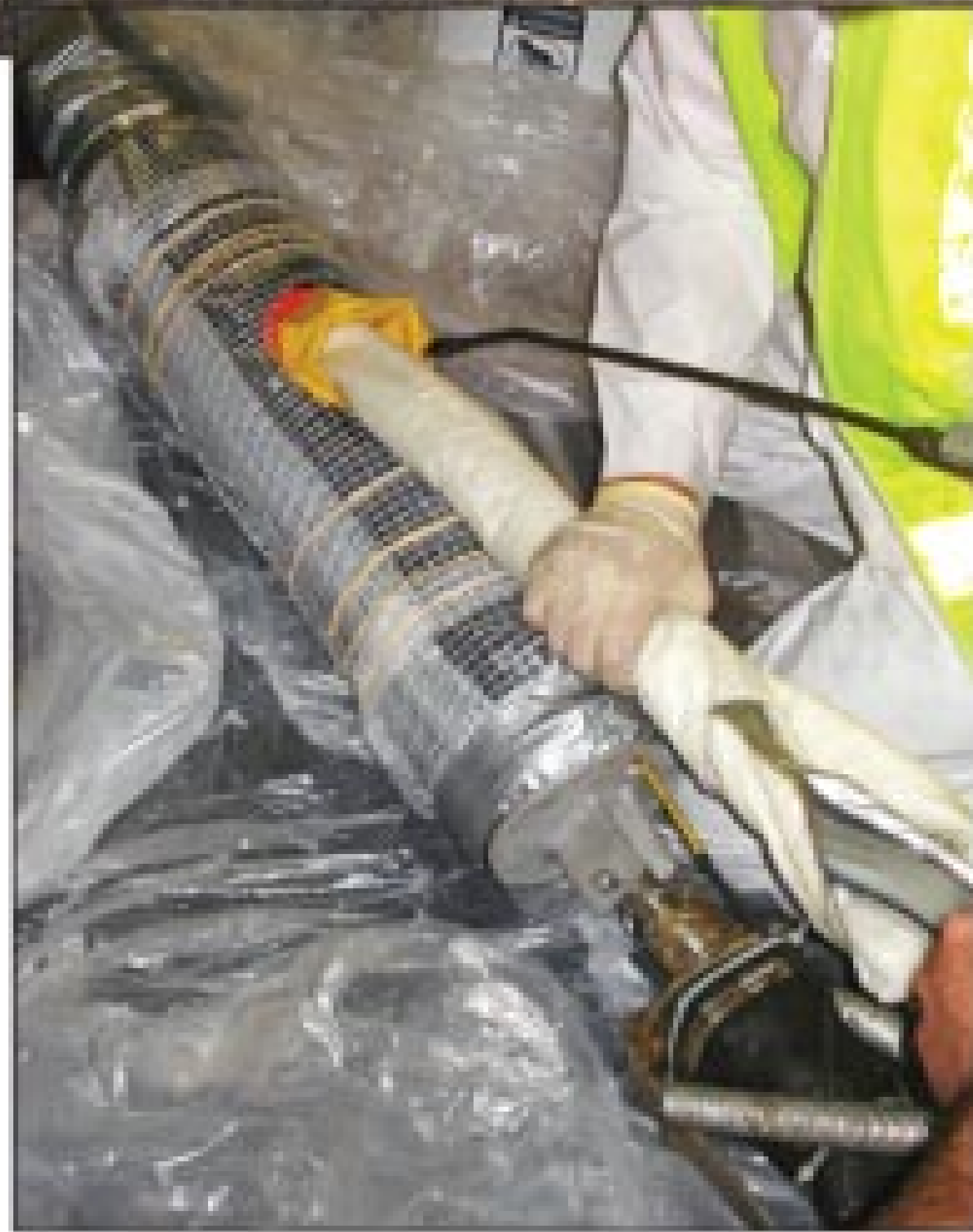
Above: Eric Sapp helps move InnerSeal lining equipment from Perma-Liner Industries down a manhole. Left: Hawaii manager Charles Woods prepares InnerSeal lining material for deployment.
