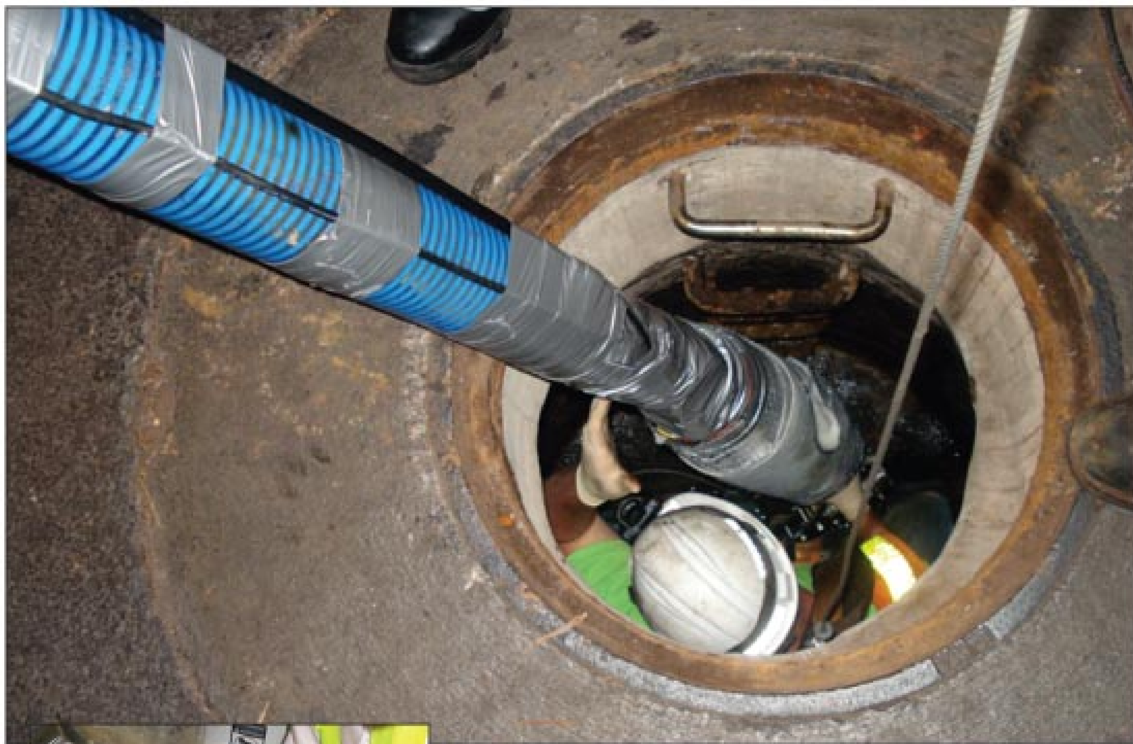
Above: Eric Sapp helps move InnerSeal lining equipment from Perma-Liner Industries down a manhole. Left: Hawaii manager Charles Woods prepares InnerSeal lining material for deployment.
