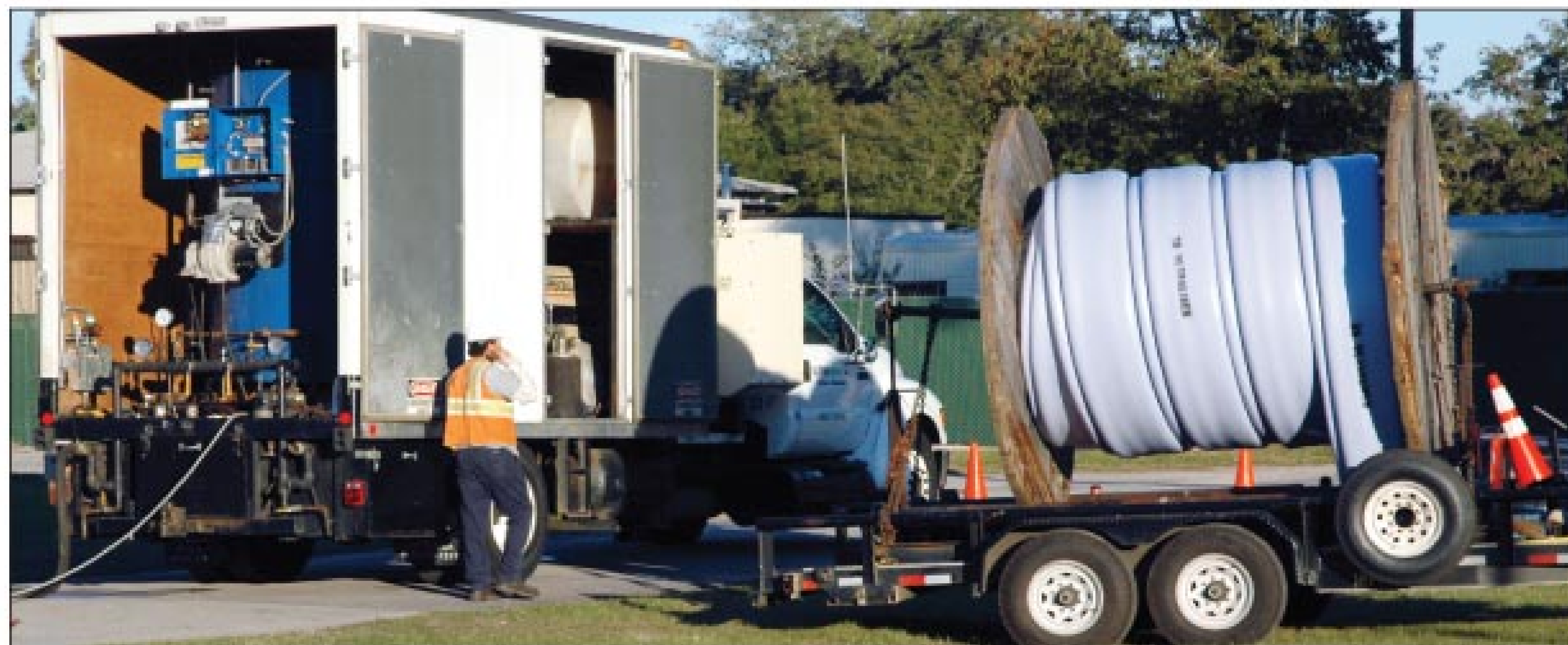
Top: The boiler truck generates steam that softens the SDR35 PVC alloy pipe, enabling it to be pulled off the spool and into the sewer. Below: Steam rises from the heated liner as workers from Engineered Lining Systems pull the head of the liner toward the manhole. (Photos courtesy of Engineered Lining Systems Inc.)
