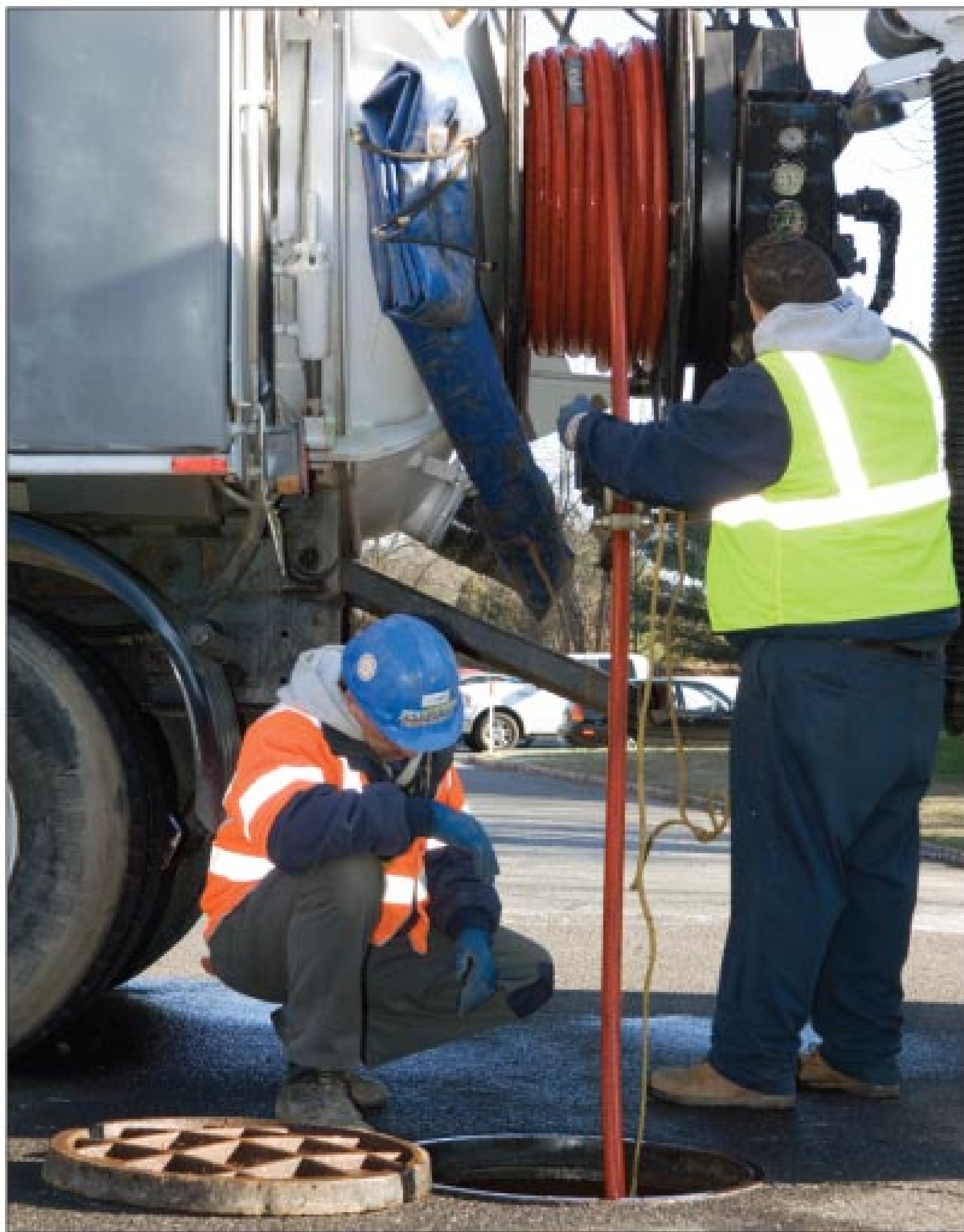
Supervisor Ray Rios and operator Darryl Stephens operate a combination truck on a sewer maintenance job.
