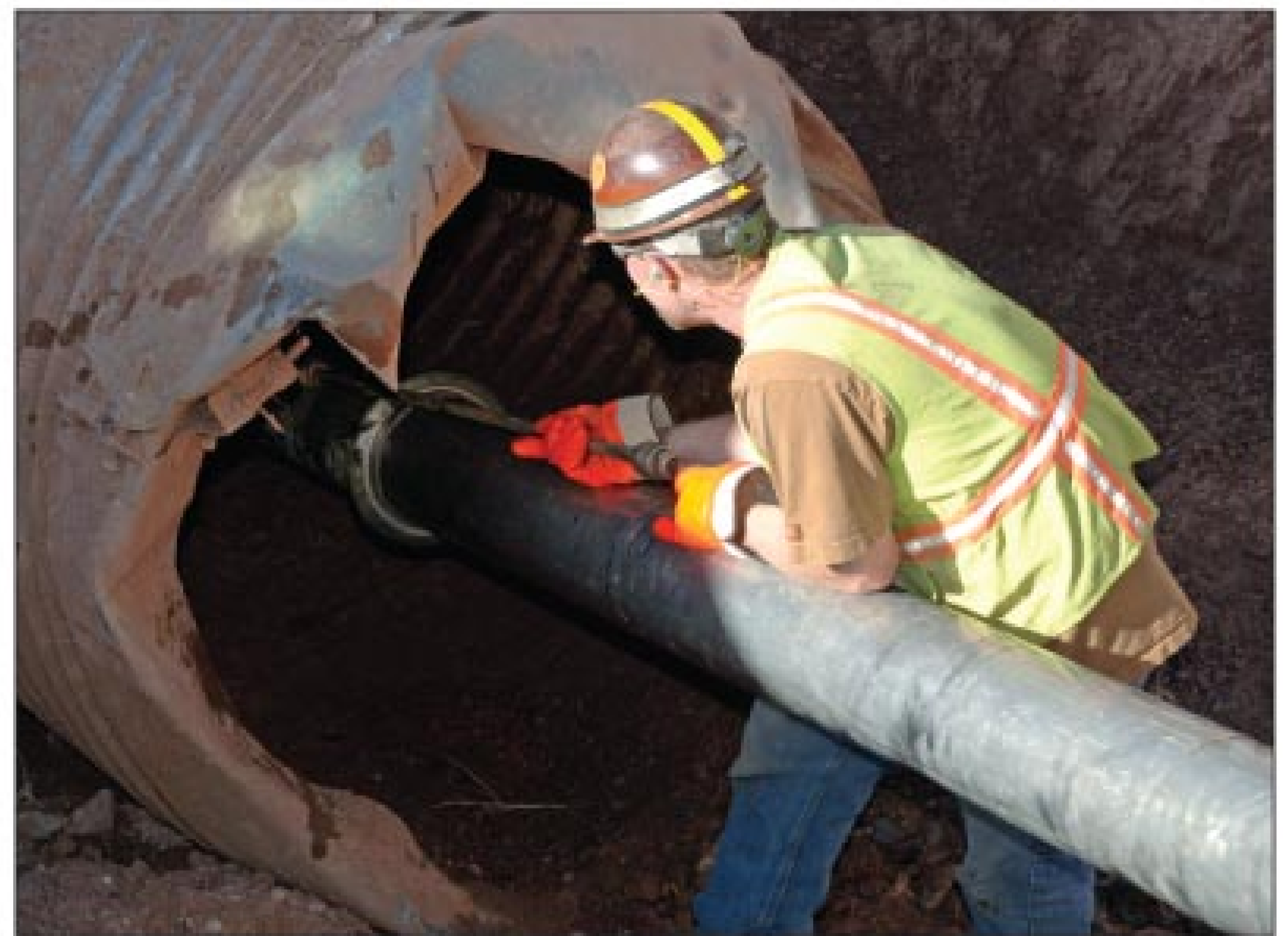
Left photo, Bob Rasnick moves an easement jetter made by Jack Doheny Supplies to an off-road work site. Right photo, Titus Larsson feeds vacuum tube into blocked culvert.
