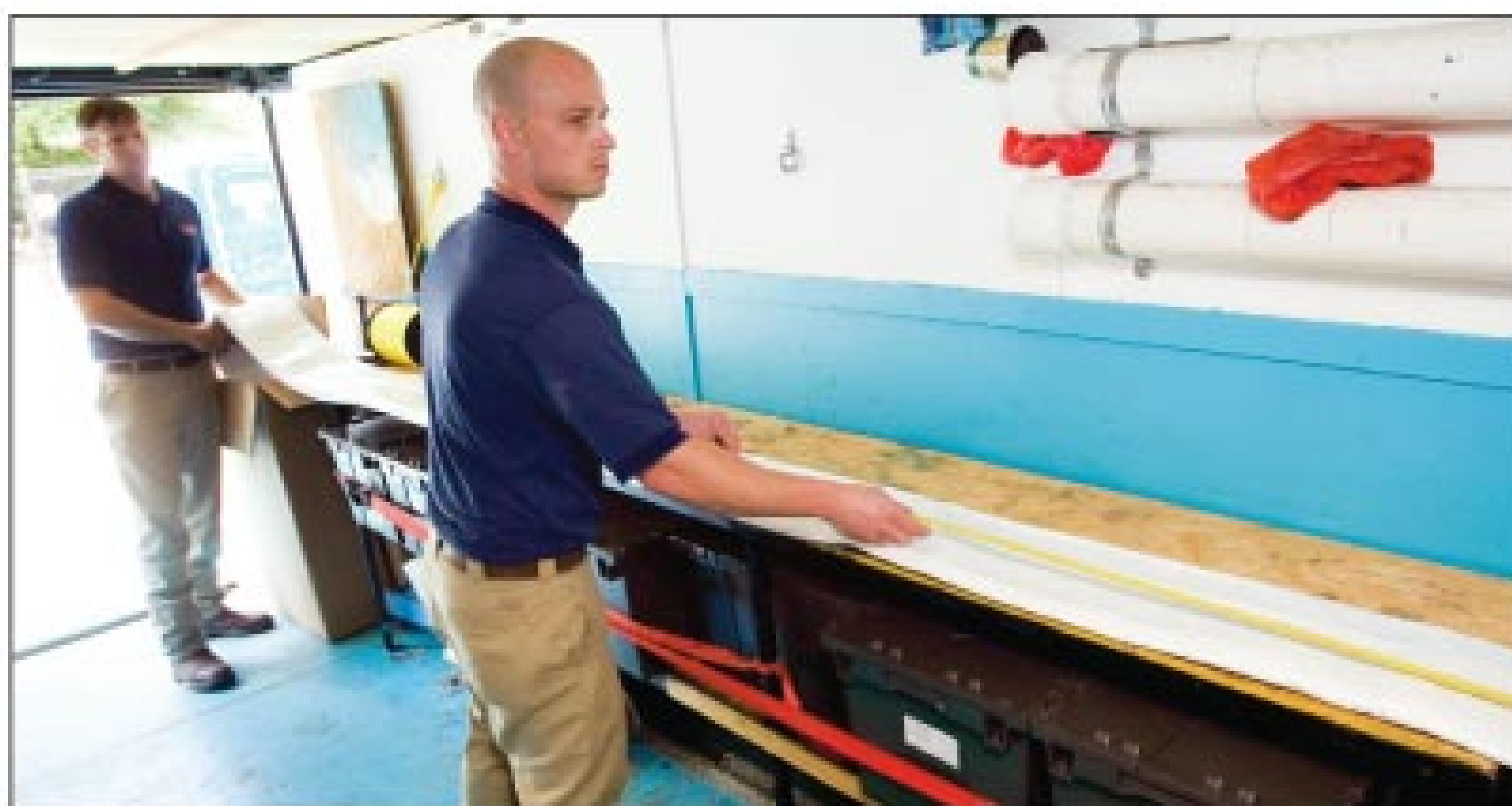
Vanlandingham (left) and technician Justin Thames prepare a new pipe liner.
