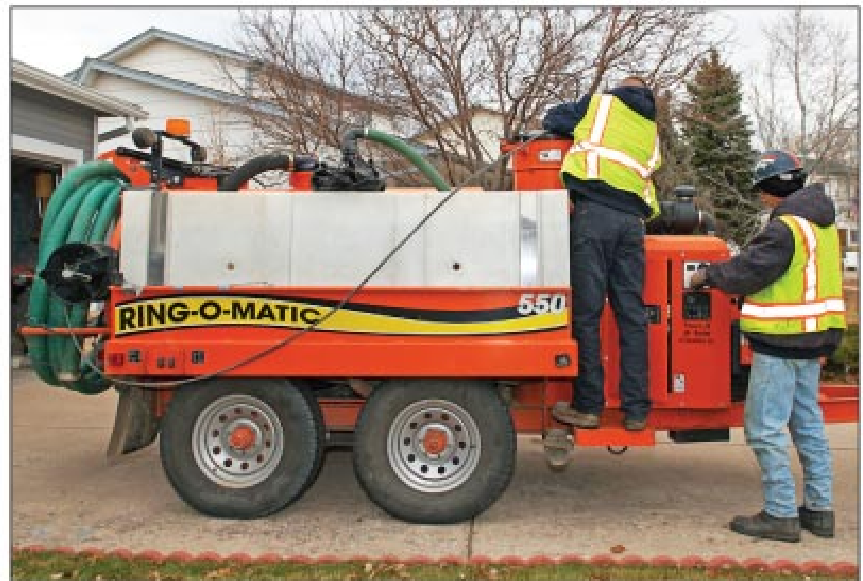
A Ring-O-Matic system provides hydroexcavation capability to Mr. Rooter of Southern Colorado.
