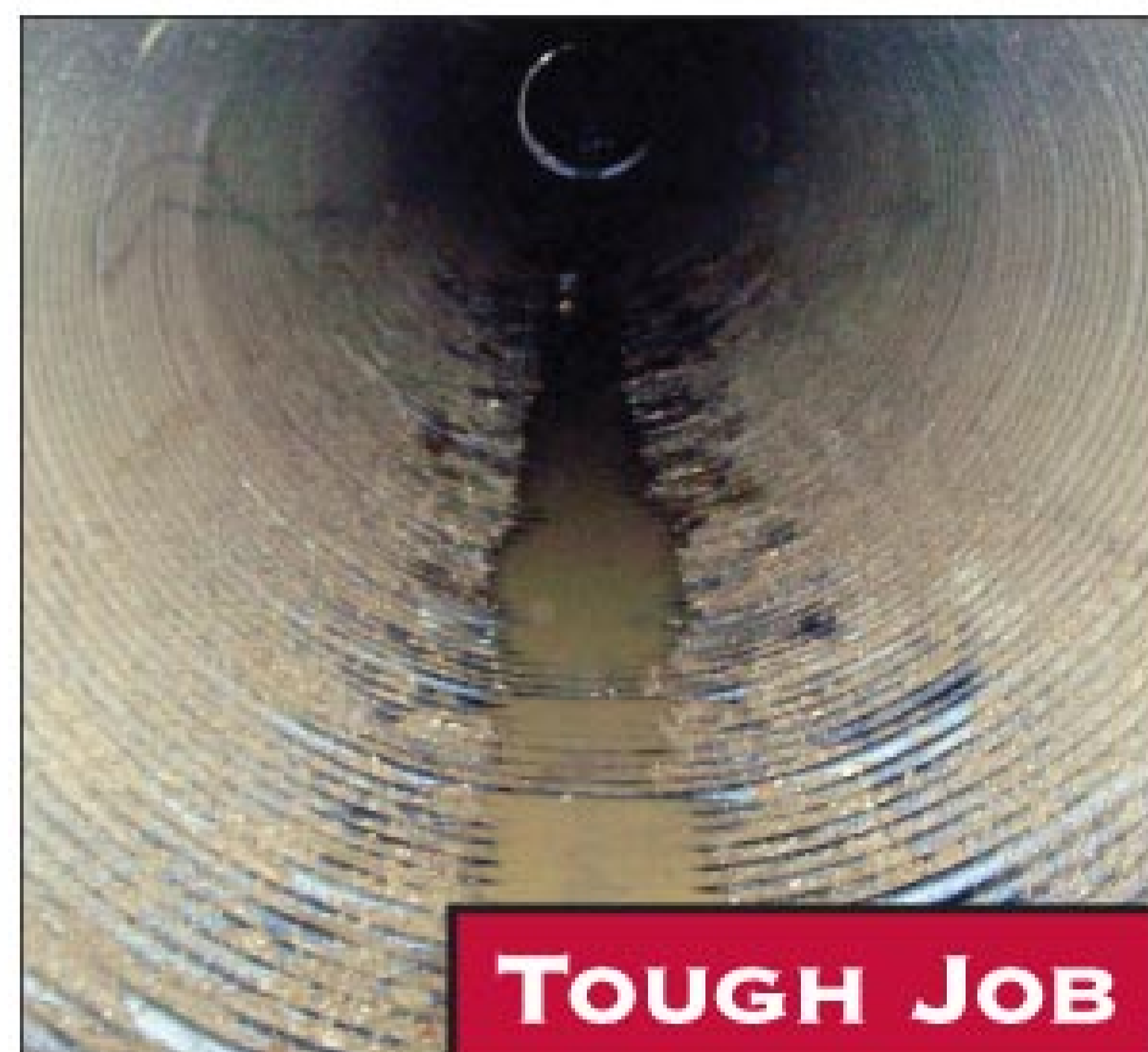
Left: Grit and organic material 3 to 4 feet deep impede flow in the 320-foot, 72-inch retention culvert. Cleaning tools are a 6-inch vacuum hose and handheld lance with standard nozzle attached to the 1/2-inch jetter hose. Right: Mission accomplished. The culvert is free of material. (Photos courtesy of Mid America Drain Service, Valley Park, Mo.)
