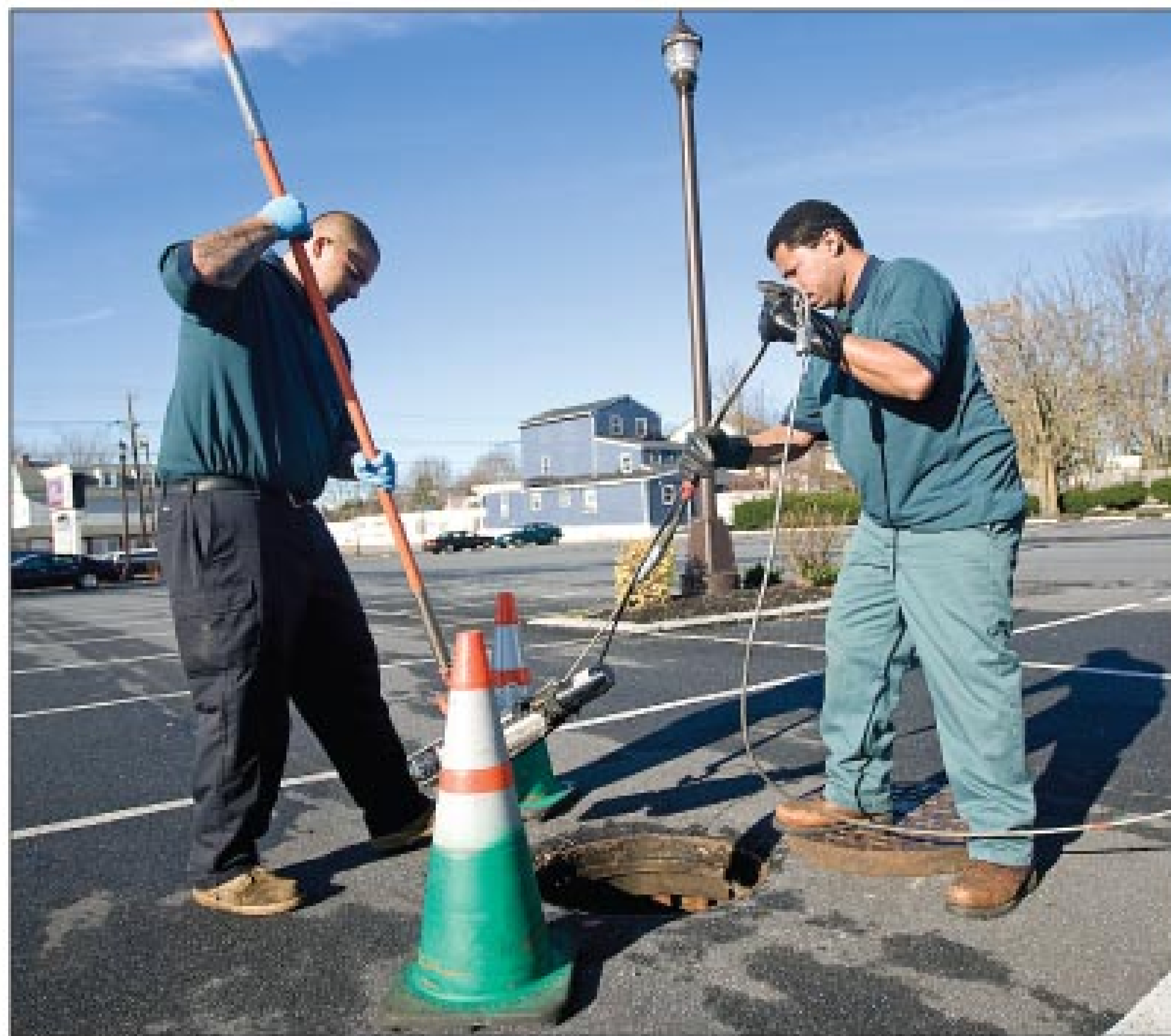
Drain Visions technicians J.R. Moore and Mike Beausil retrieve an inspection camera after a job in Blackwood, N.J.
