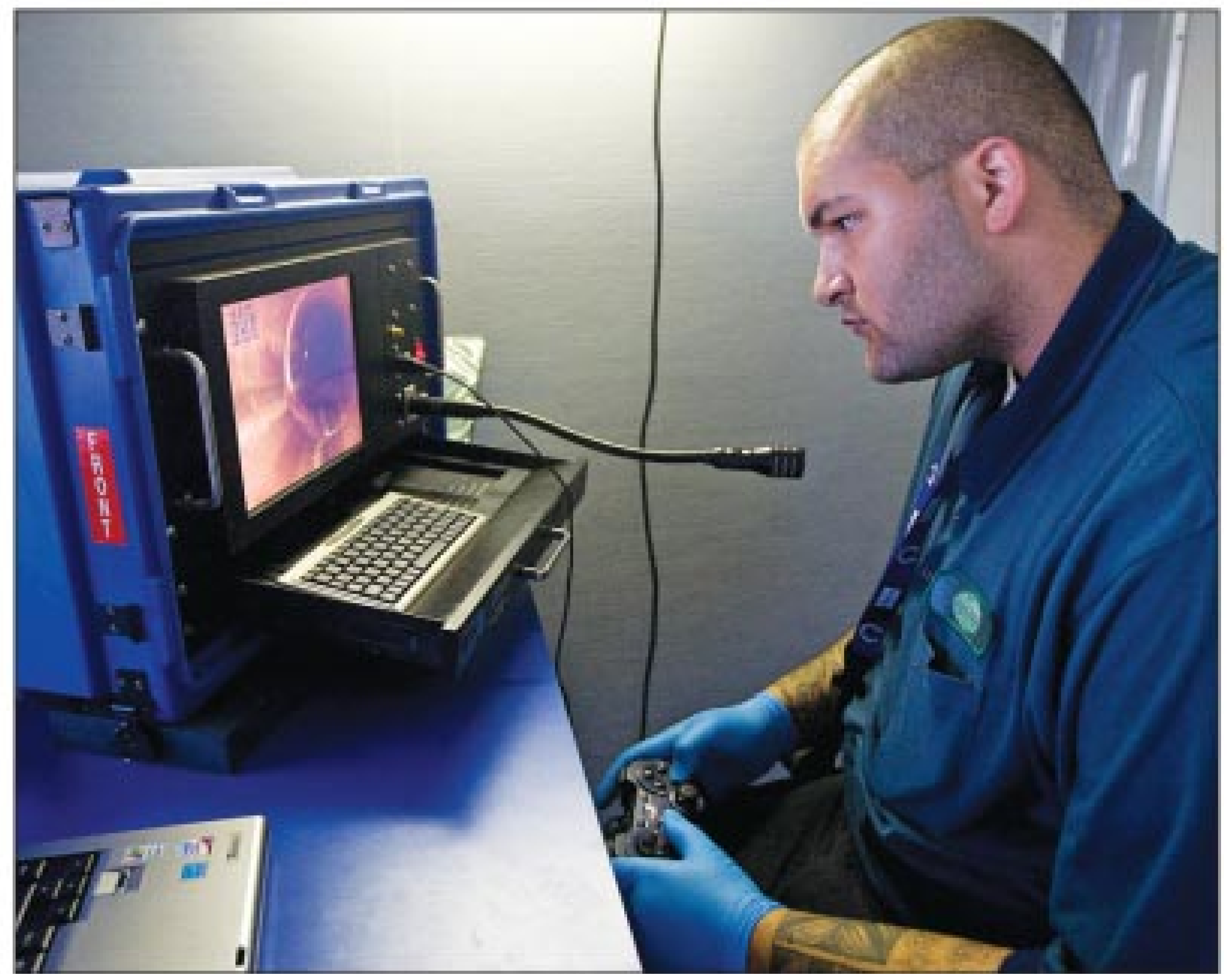
J.R. Moore conducts and observes a mainline inspection with a K2 portable inspection system from CUES Inc.
