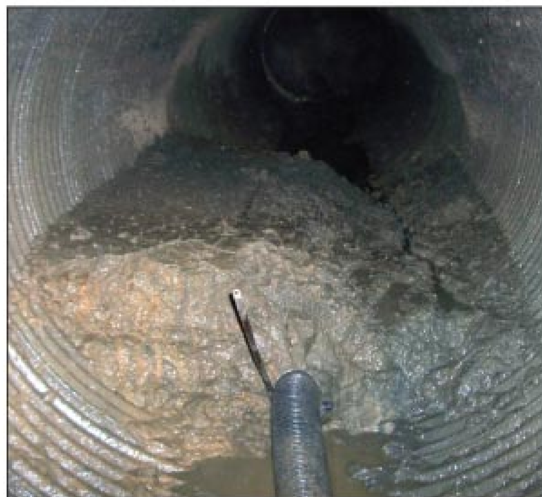
Left: Grit and organic material 3 to 4 feet deep impede flow in the 320-foot, 72-inch retention culvert. Cleaning tools are a 6-inch vacuum hose and handheld lance with standard nozzle attached to the 1/2-inch jetter hose. Right: Mission accomplished. The culvert is free of material. (Photos courtesy of Mid America Drain Service, Valley Park, Mo.)
