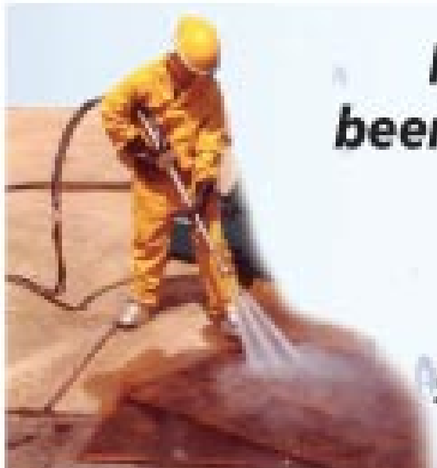
Water Blasting Dump Gun used for cleaning & surface preparation
