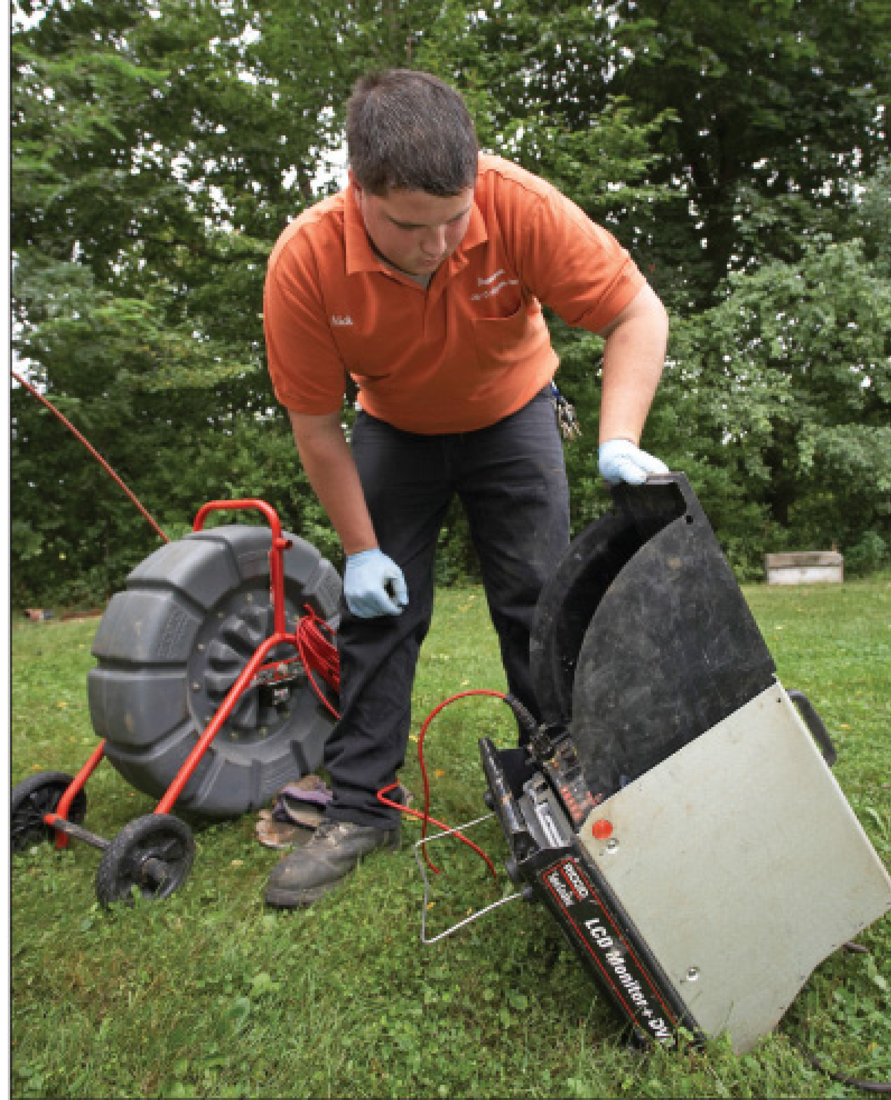
Service technician Nicholas St. Croix at the monitor on a lateral inspection job.
