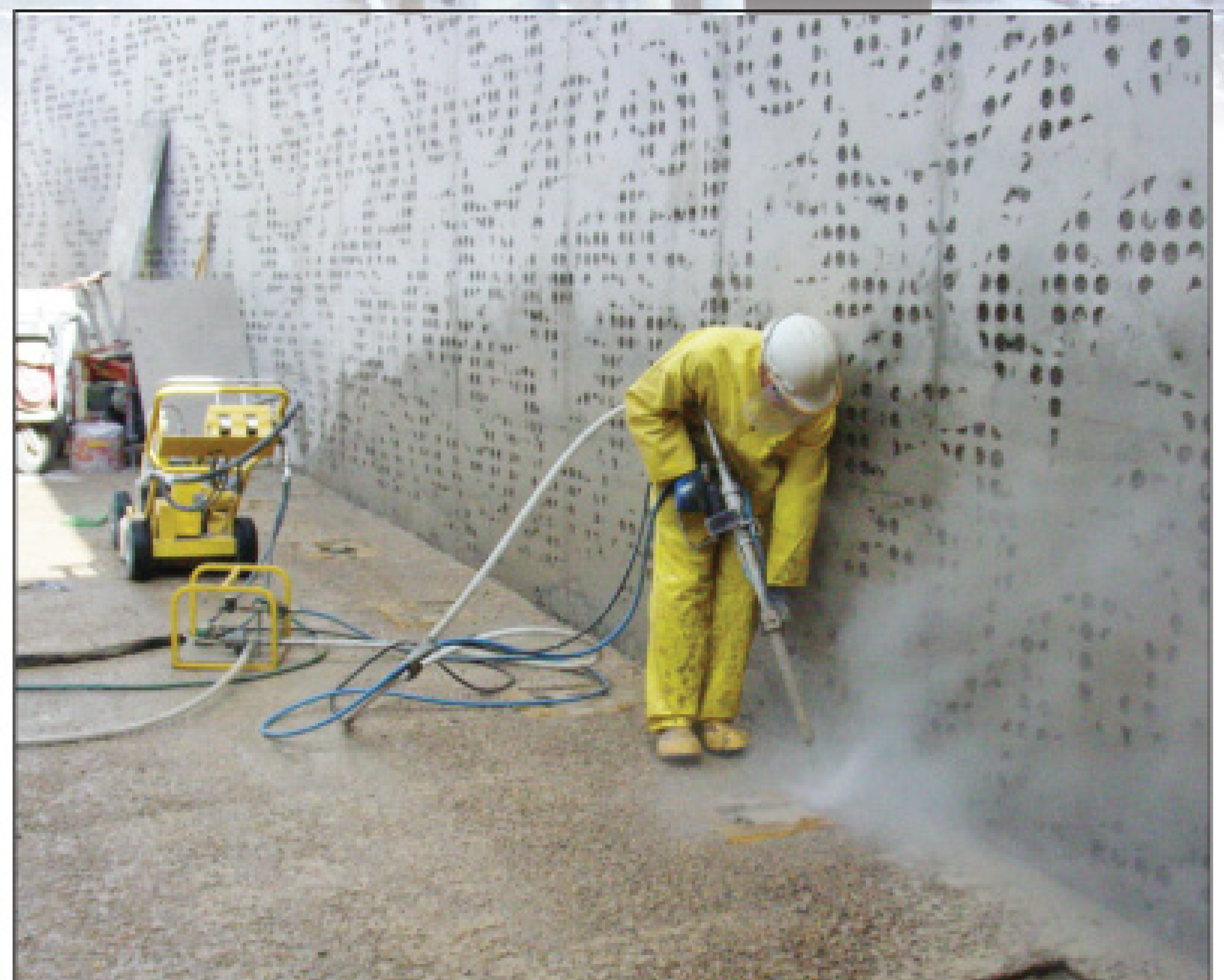
Midwest Mobile Waterjet used its work tools to create a unique design on the walls of the Walker Art Center in Minneapolis, Minn. (Photos courtesy of Brian Gleeson)
