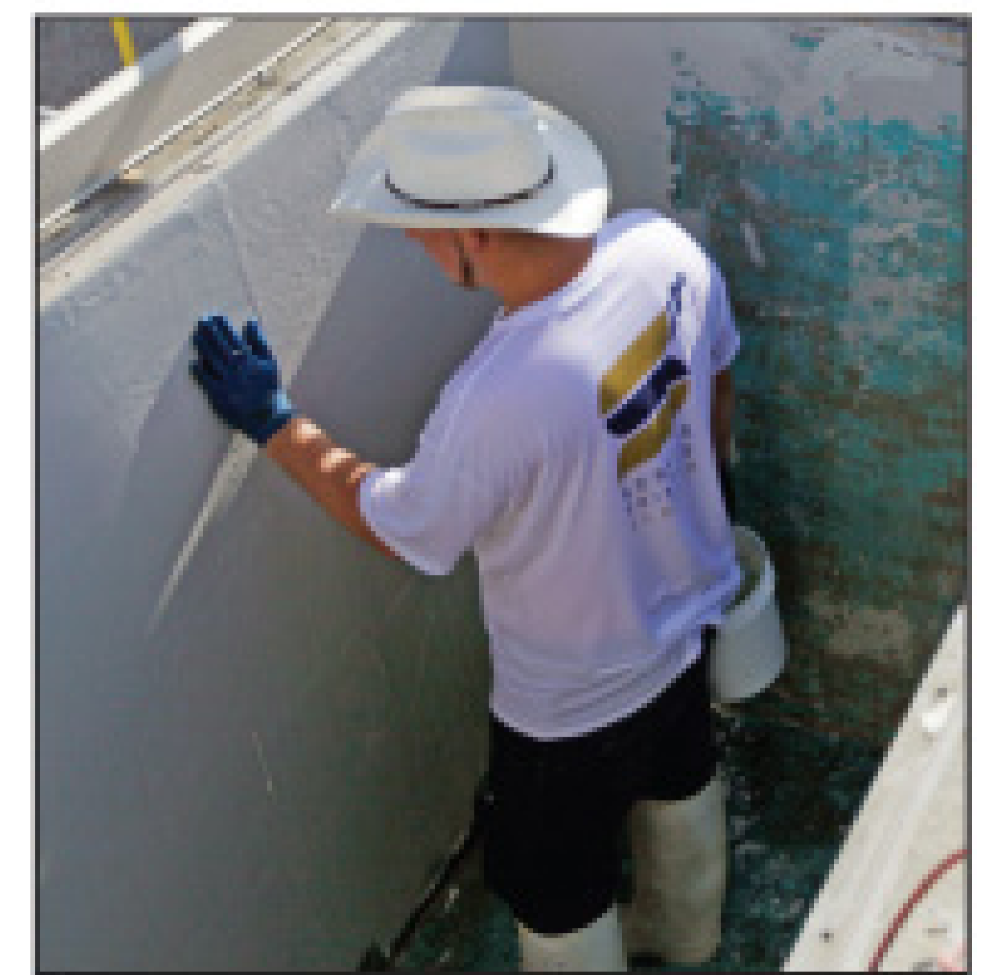
Service Painting specialties include stripping off old industrial coatings with high-pressure water and then repainting with long-lasting epoxy and other paint formulations.
