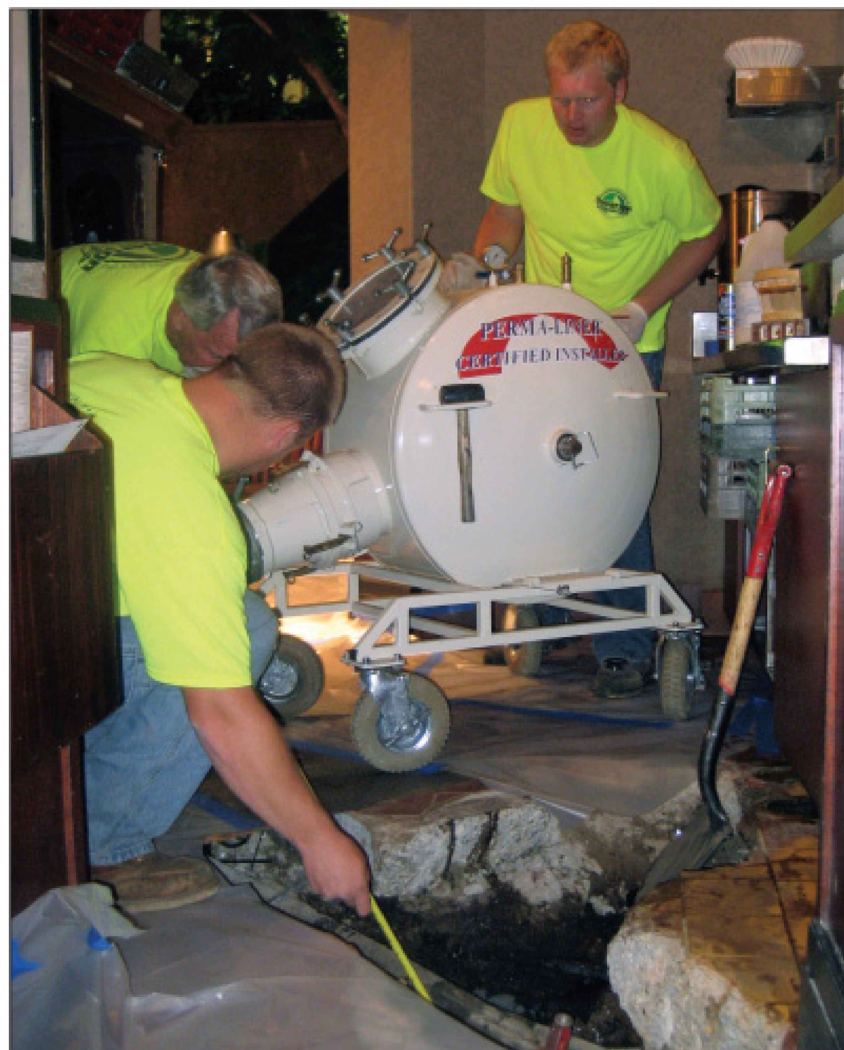
Troy Ouverson (standing) and Doug Ouverson position the air inversion tank as Scott Veal measures the distance from the tank to the pipe about to be lined. (Photos from Troy Ouverson)
