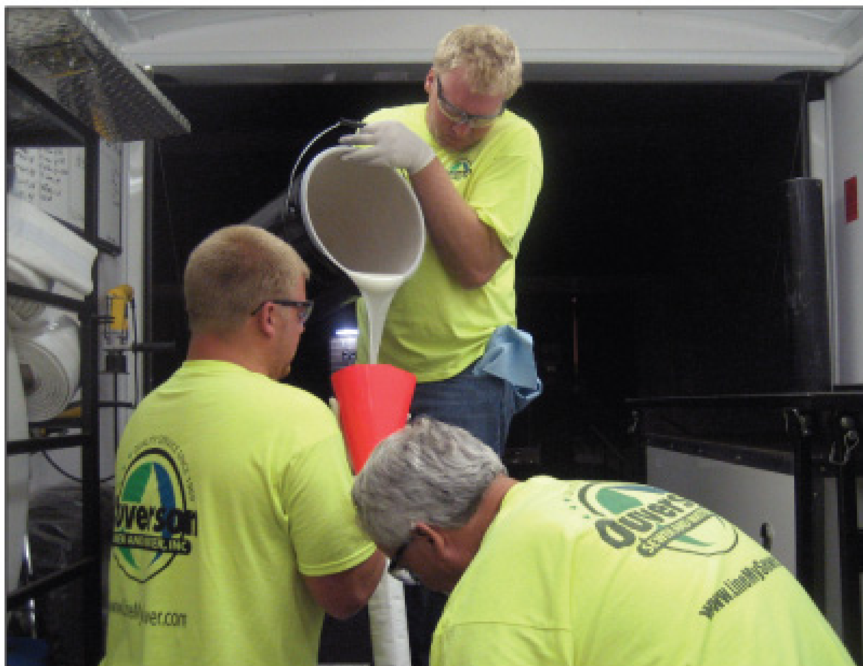
Troy Ouverson pours resin into a cone to begin the wetting-out process. Scott Veal holds the cone and Doug Ouverson assists him.
