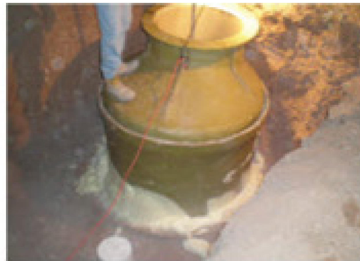
THE CONE IS REMOVED AND THE COMPOSITE IS INSERTED
