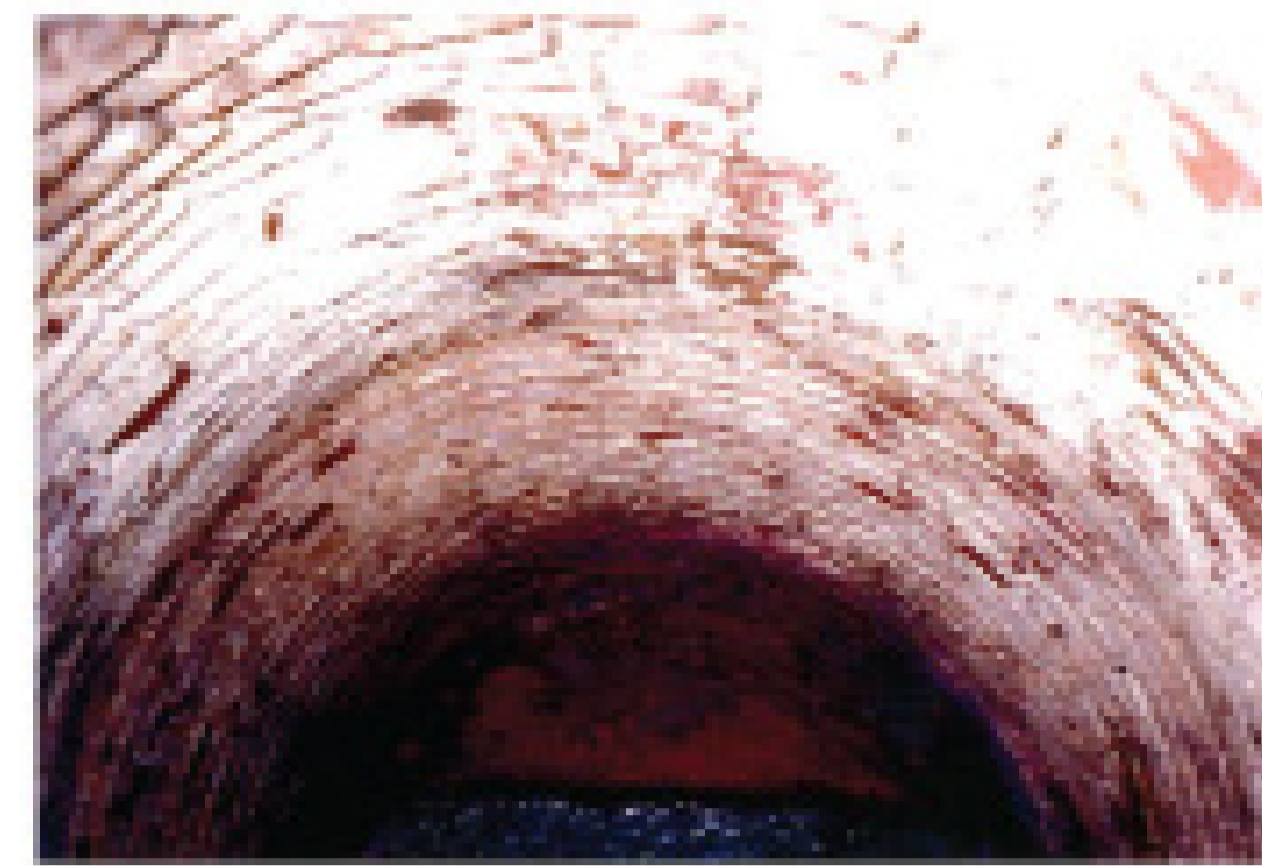
BRICK MANHOLE BEFORE REHABILITATION
