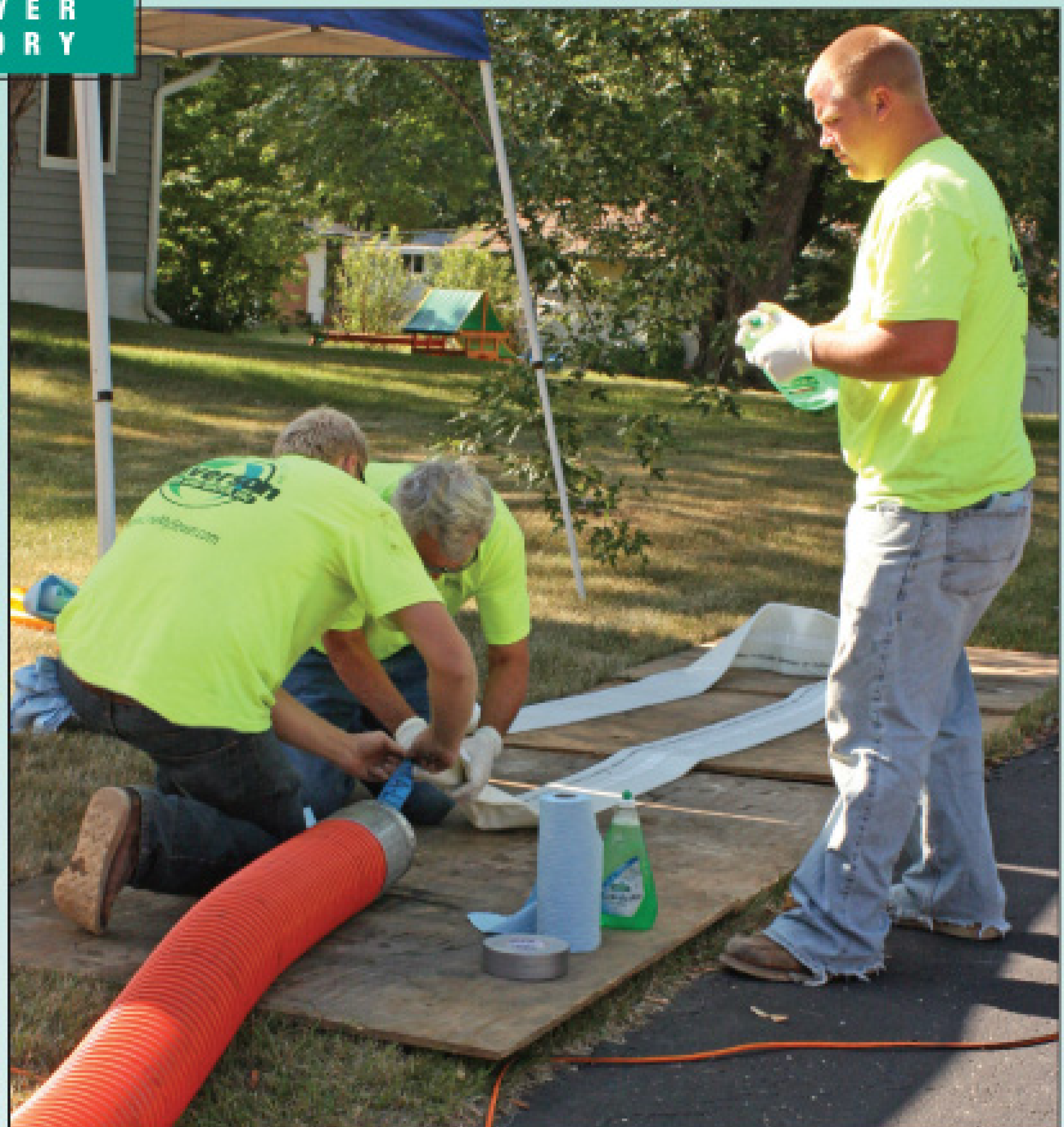
Left Photo: Troy Ouverson, shown on a pipe lining job, leads a company that has found success by diversifying its services. Right photo, from left, Troy Ouverson, Doug Ouverson and Scott Veal lubricating a liner with soap to make it easier to invert through the sewer pipe. (Photography by Mary R. Christen)
