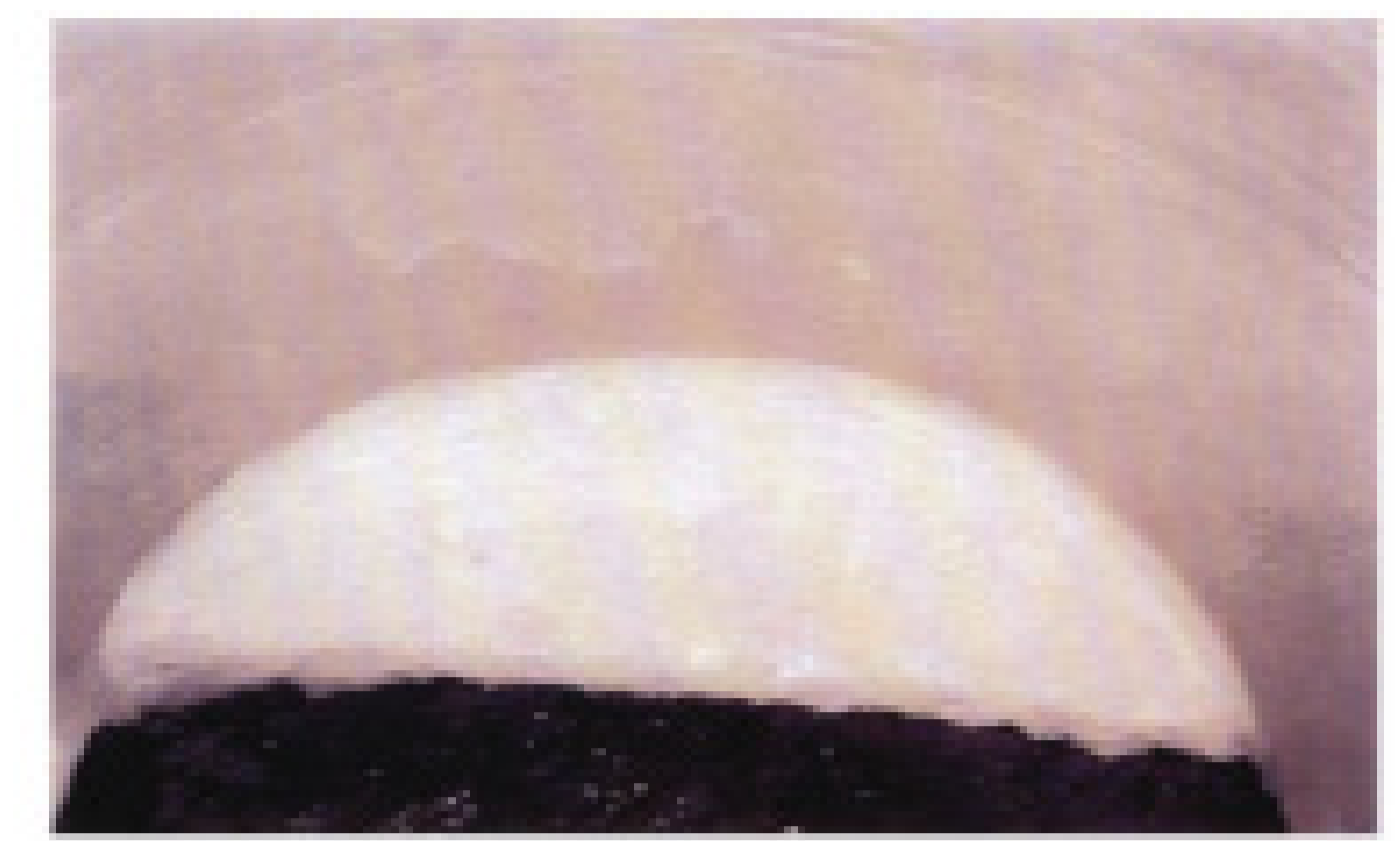
BRICK MANHOLE AFTER REHABILITATION
