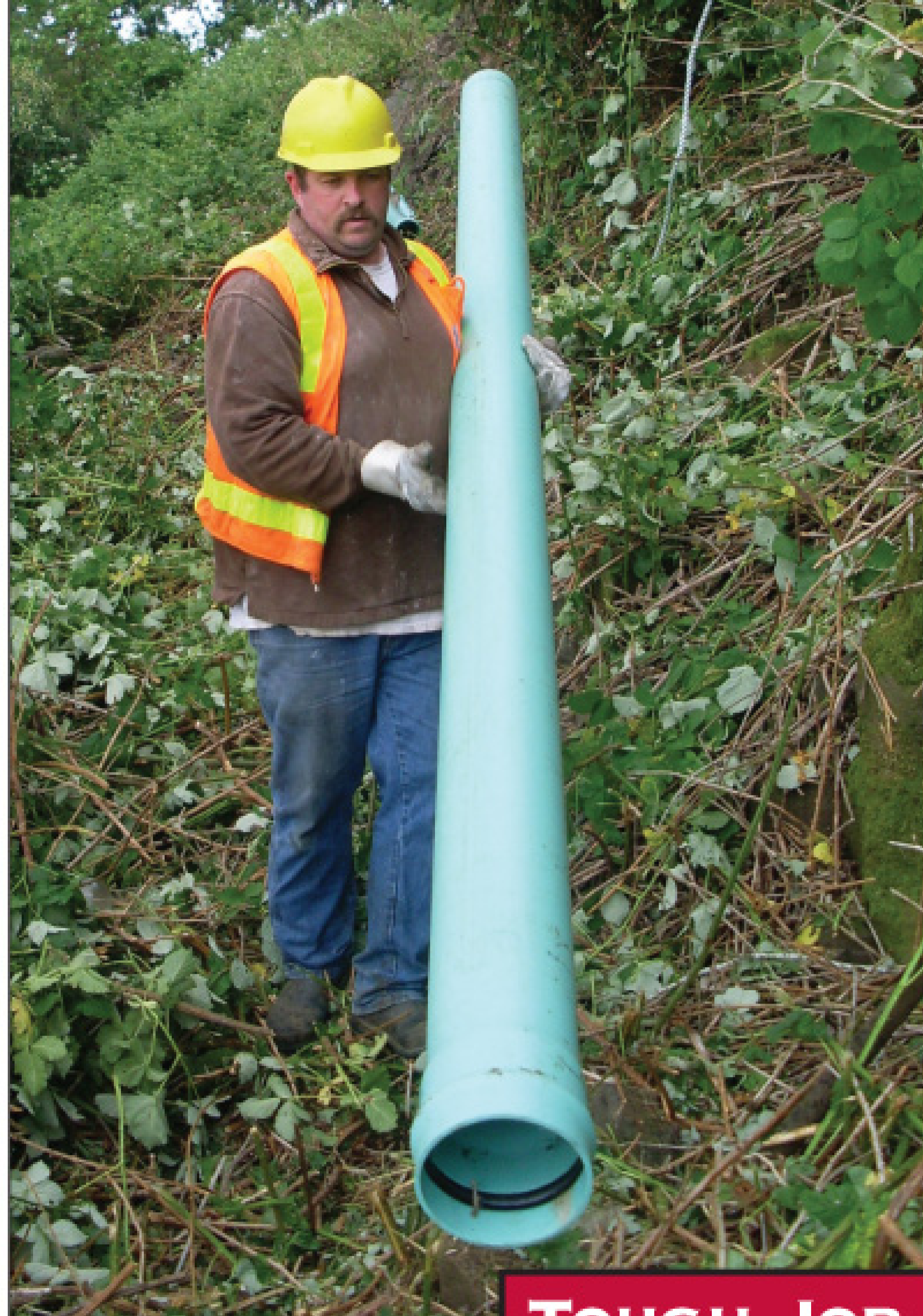
Certified lining installer Steve Neal carries a length of bypass pipe down the side of a cliff for placement. (Photos courtesy of Zwald Industrial Services.)
