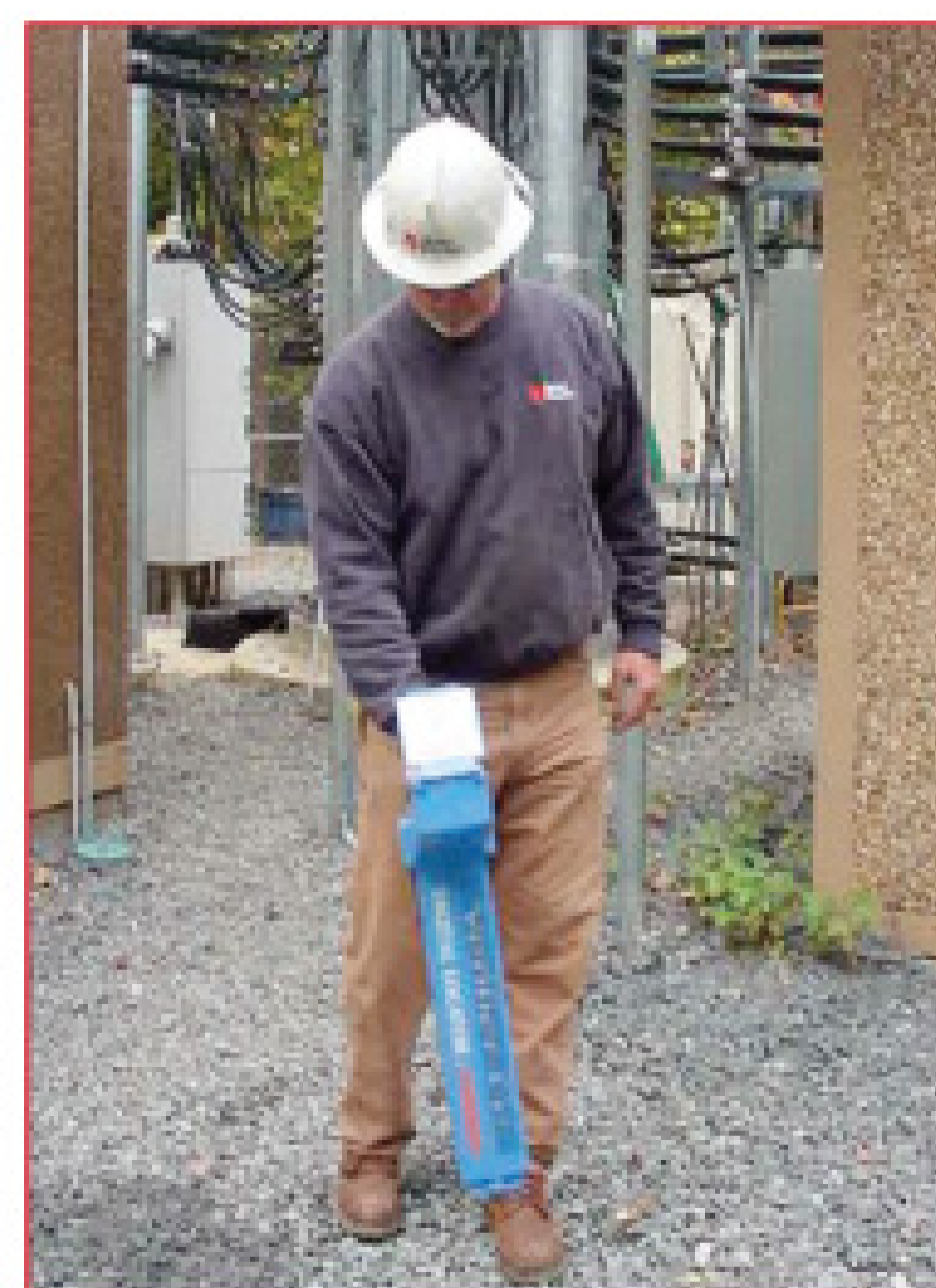
A locator is used at an electrical substation as part of a project addition at the site. (Photos courtesy of McLaughlin)
