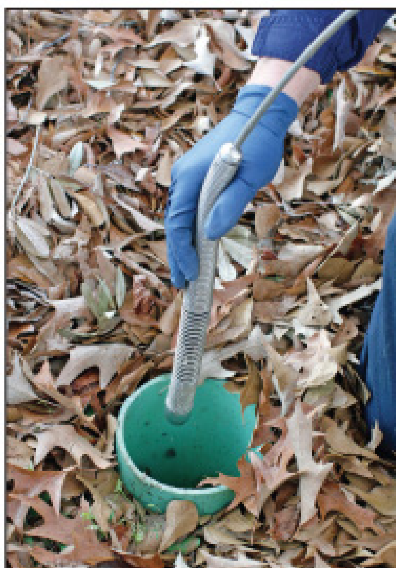
A push camera is deployed for a residential inspection job.
