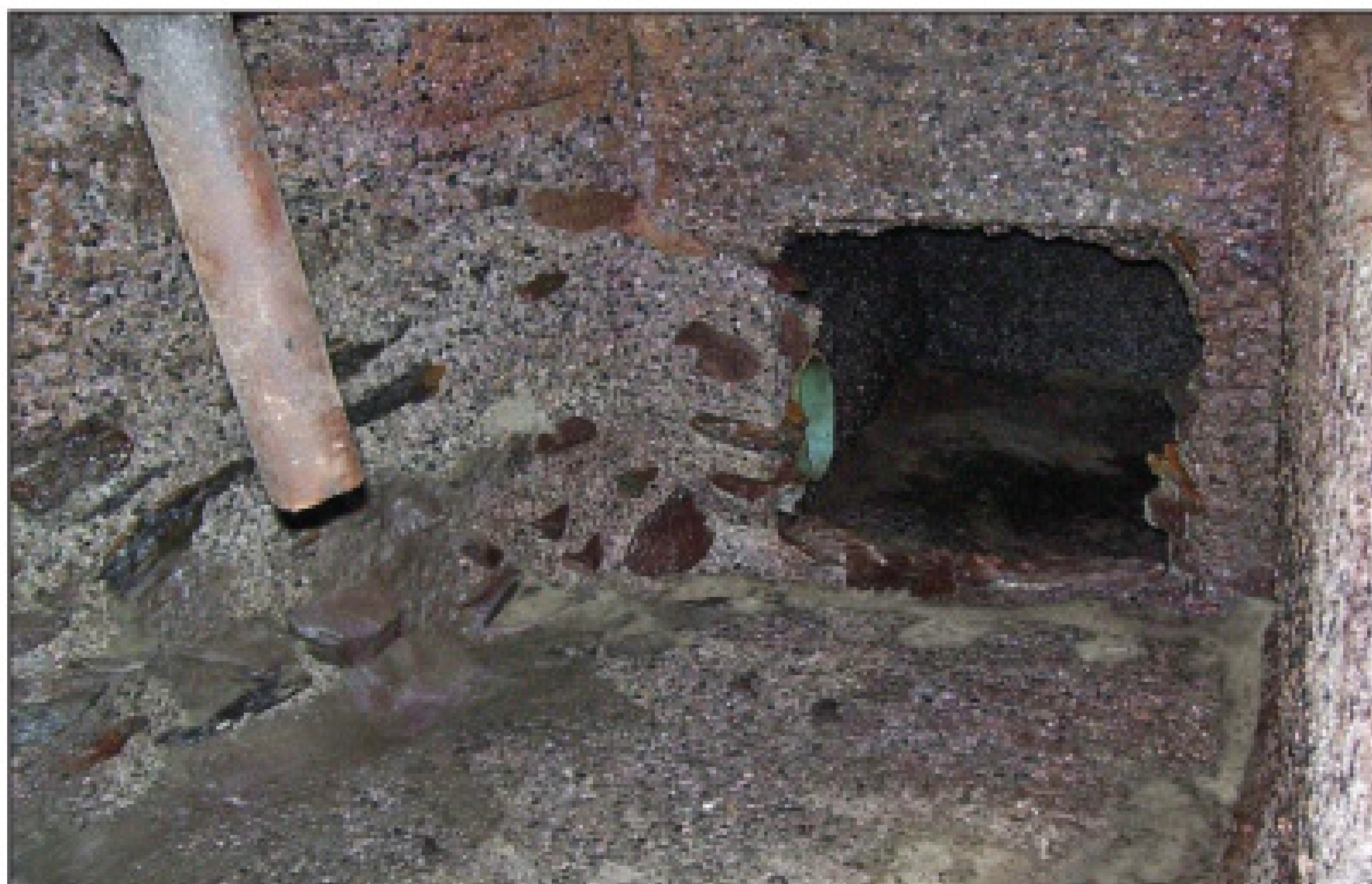
Men and hoses went back and forth between the outside and inside tanks through this 2-foot-square opening.
