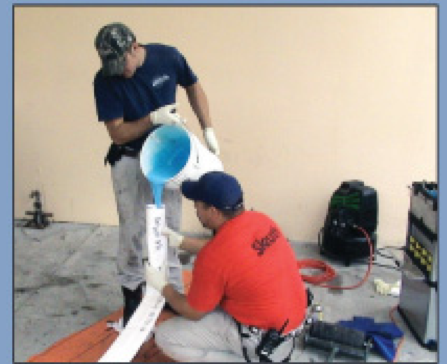
Josh Miller pours mixed two-part epoxy into a felt liner held by Alfonso Rodriguez.
