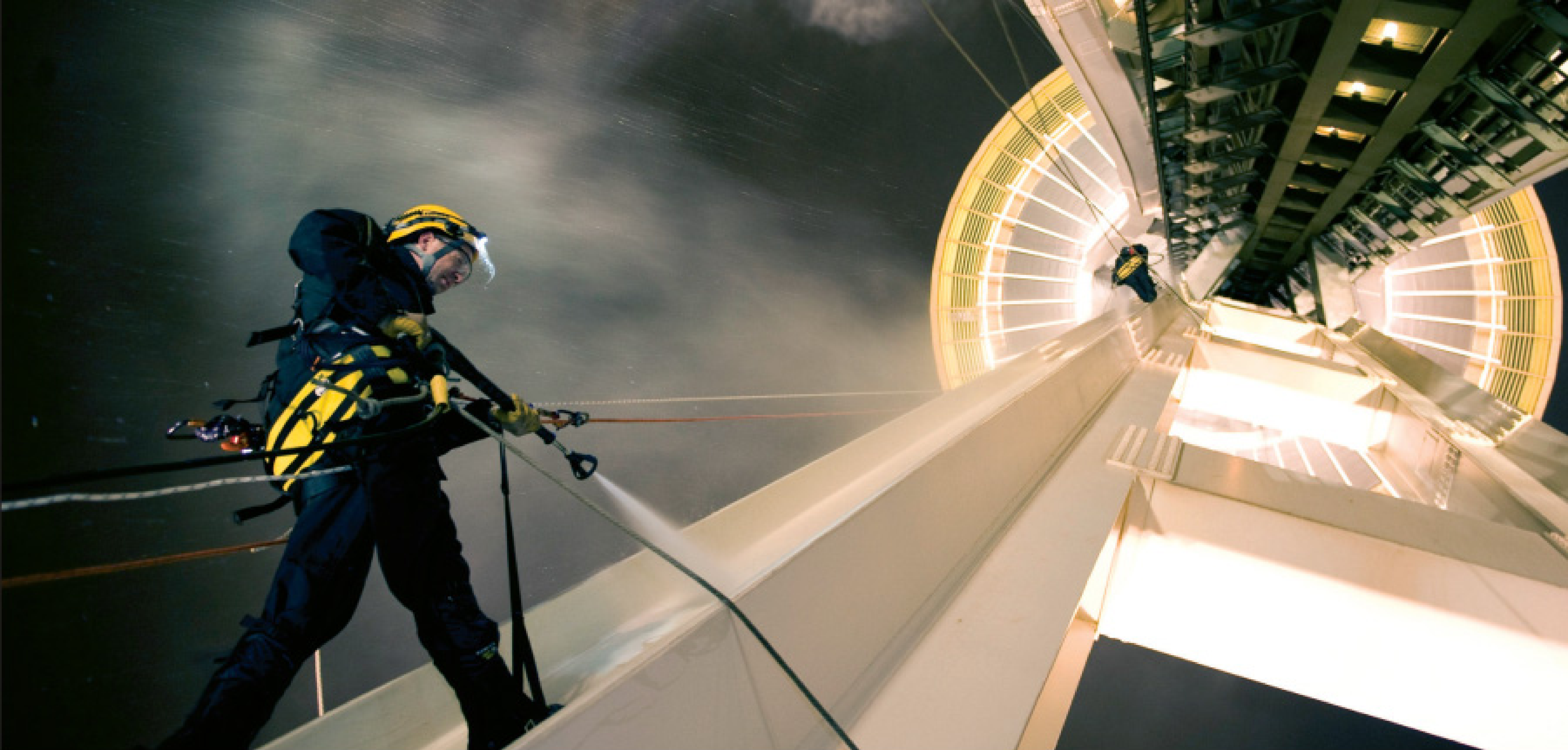
Plain water heated to 194 degrees Fahrenheit removes grime from air pollution, algae, bird droppings and elevator grease without damaging paint.
