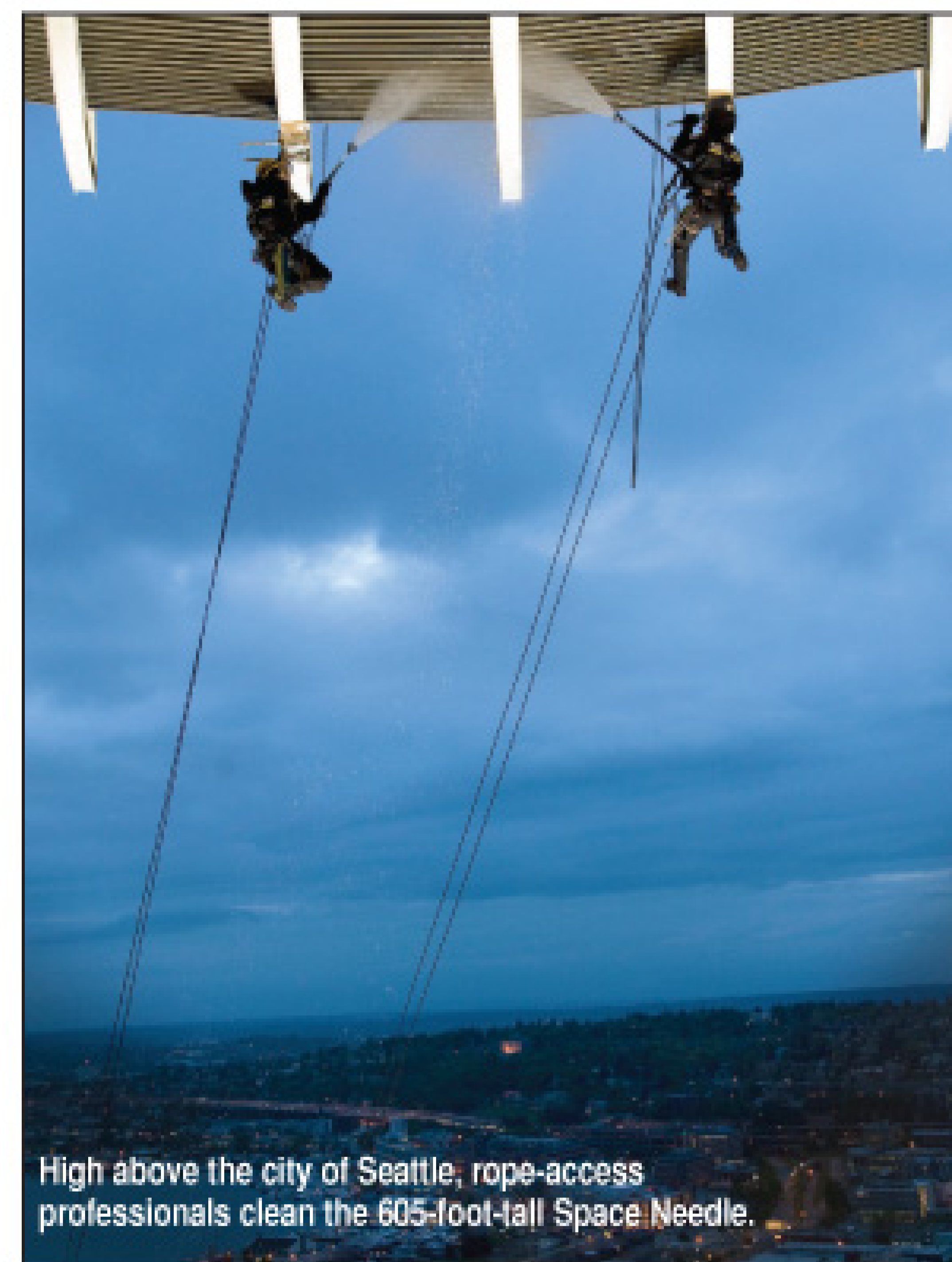
Plain water heated to 194 degrees Fahrenheit removes grime from air pollution, algae, bird droppings and elevator grease without damaging paint.
