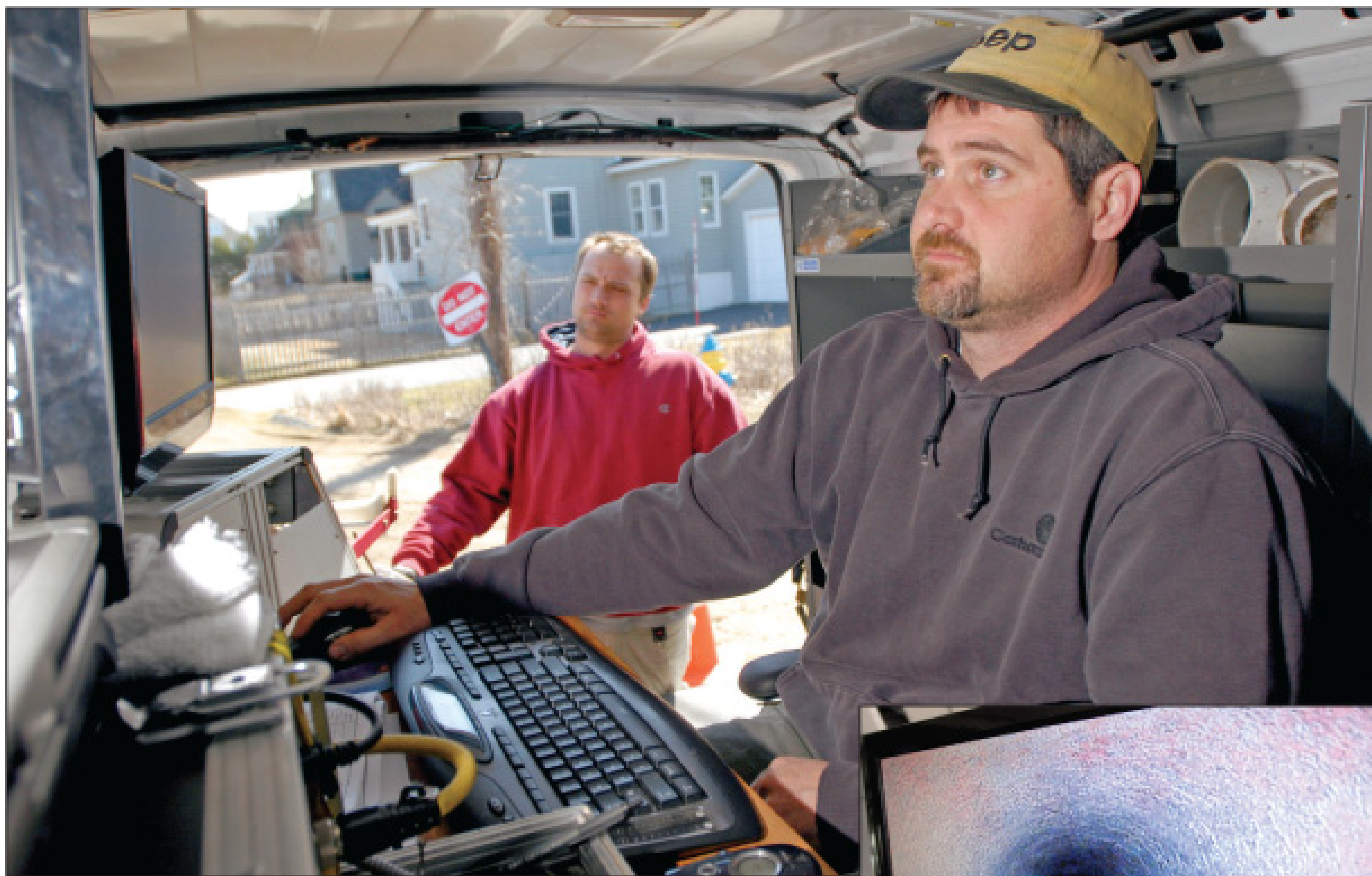
Company owner Greg Goan operates an EnviroSight robotic crawler from inside a van during an inspection in Kennebunk, Maine.
