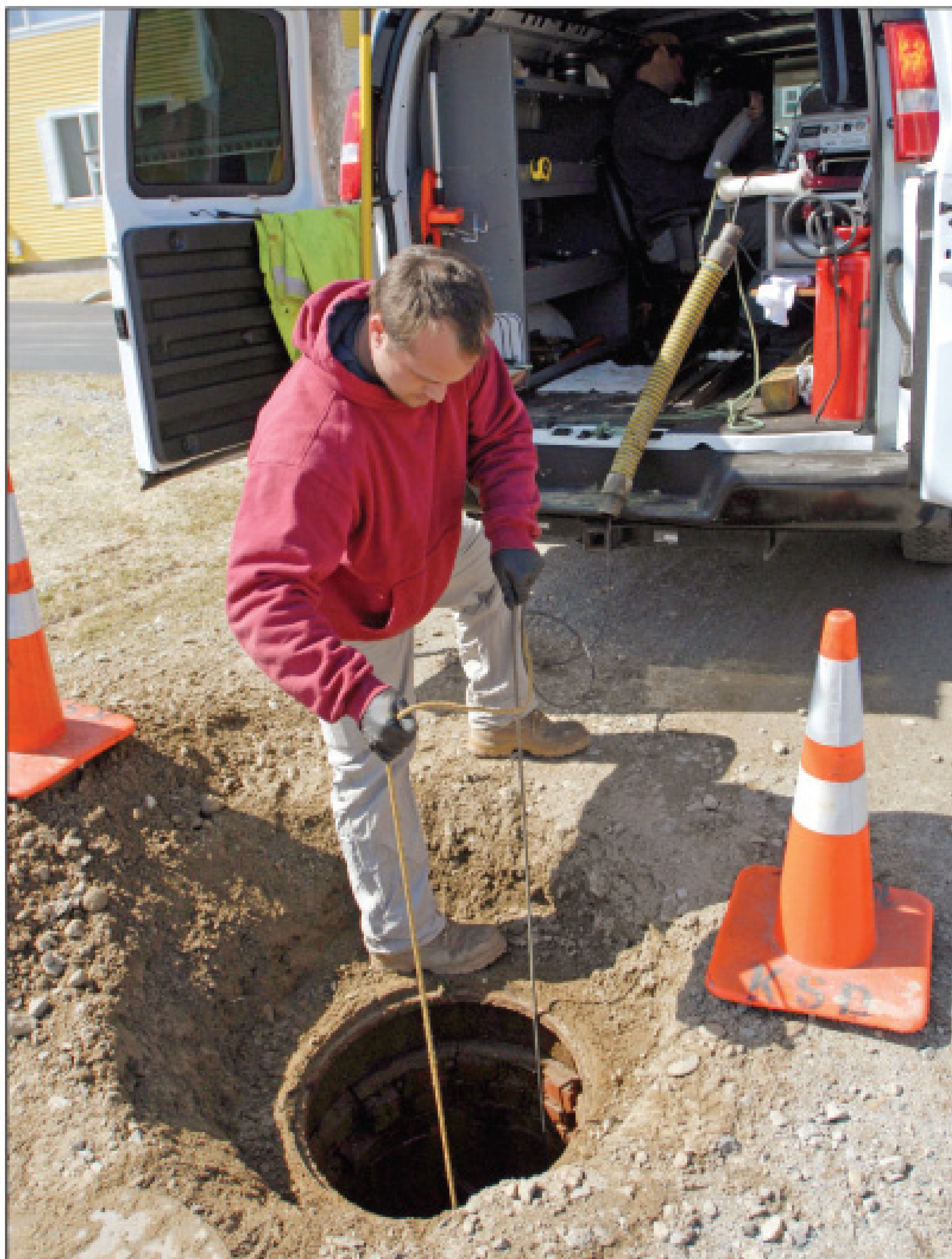
Keith Emory lowers an EnviroSight camera and robotic crawler into a sewer line during an inspection.
