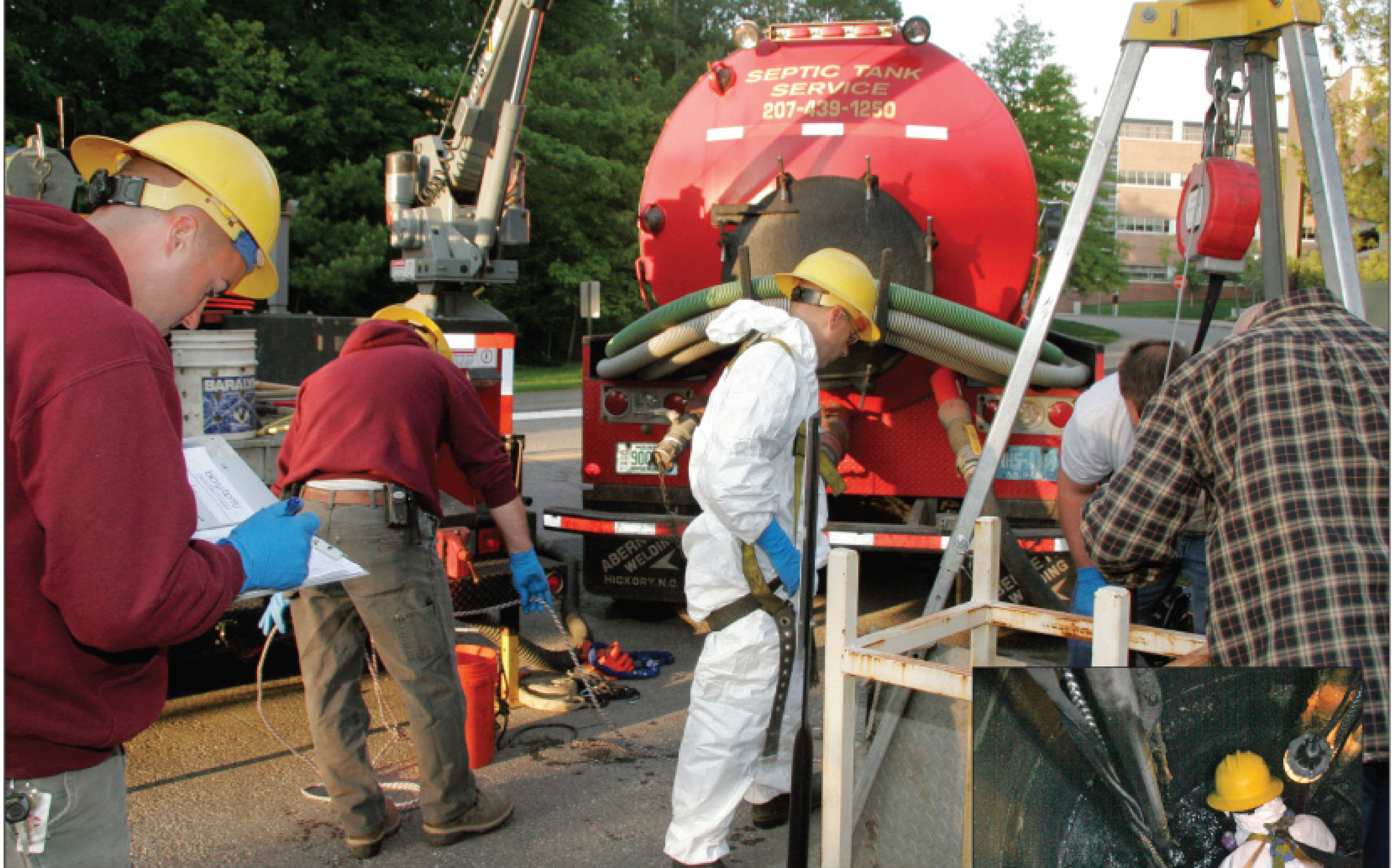
Jason Beauregard, left, of Sturgeon Creek Enterprises, keeps a federal report of gas levels while Hunter Smigelski works in the confined space. Second from left is Sturgeon Creek owner Mike Dupuis, and to his right is Dan Flint. At the far right, Bill Morgridge, owner of L.W. Morgridge & Son, and employee Matt Lizotte monitor Smigelski's progress in the tank.
