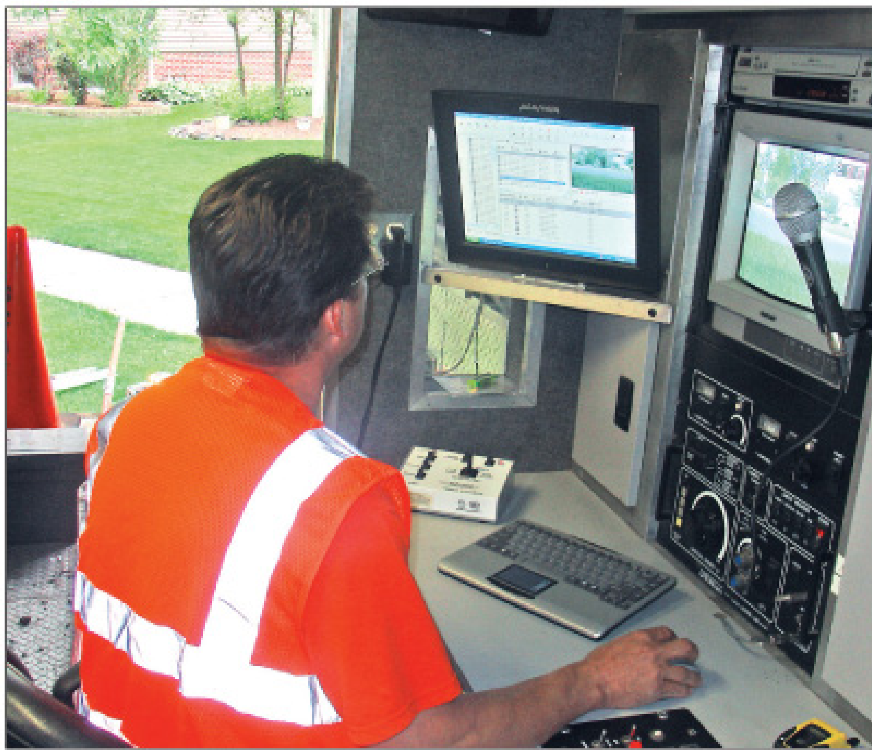
An A-K Underground technician monitors a video inspection. (Photo courtesy of A-K Underground)
