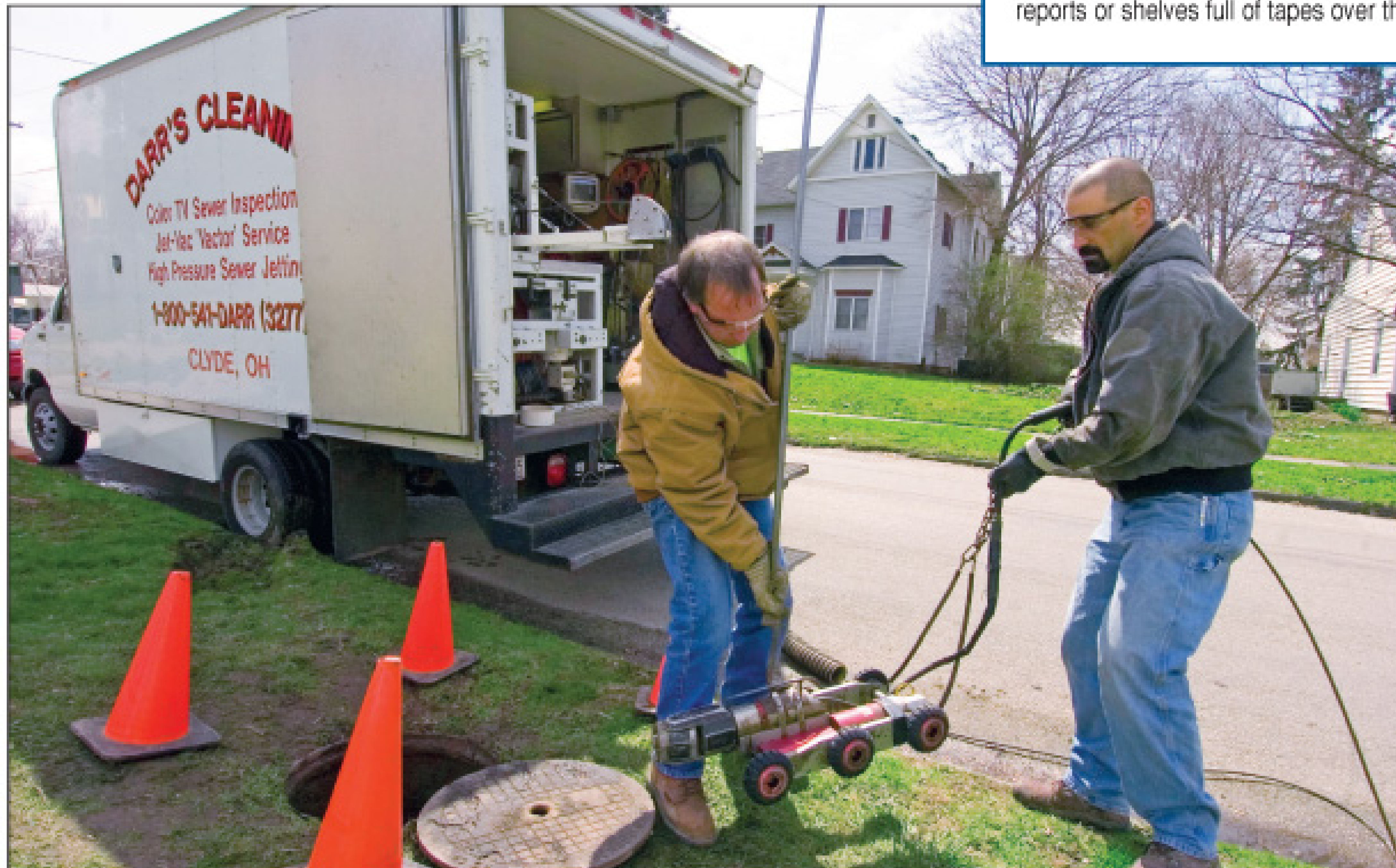
Above, Harold Darr (left) talks to his son and current owner Bernie Darr after cleaning out a farmer’s septic tank using the company’s 2006 International PayStar 5600 vacuum truck built by Precision Tank & Equipment. At left, Roger Darr (left) co-owner of Darr’s Cleaning, and technician Steve Frate lower a tractor unit with a pan-and-tilt camera from Aries Industries Inc.
