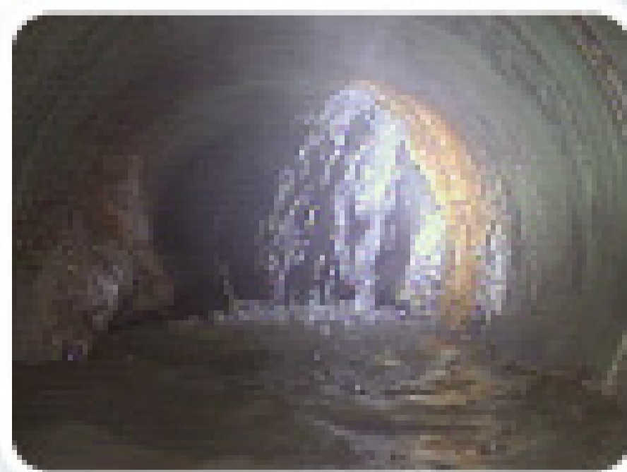
Gushing Infiltration
