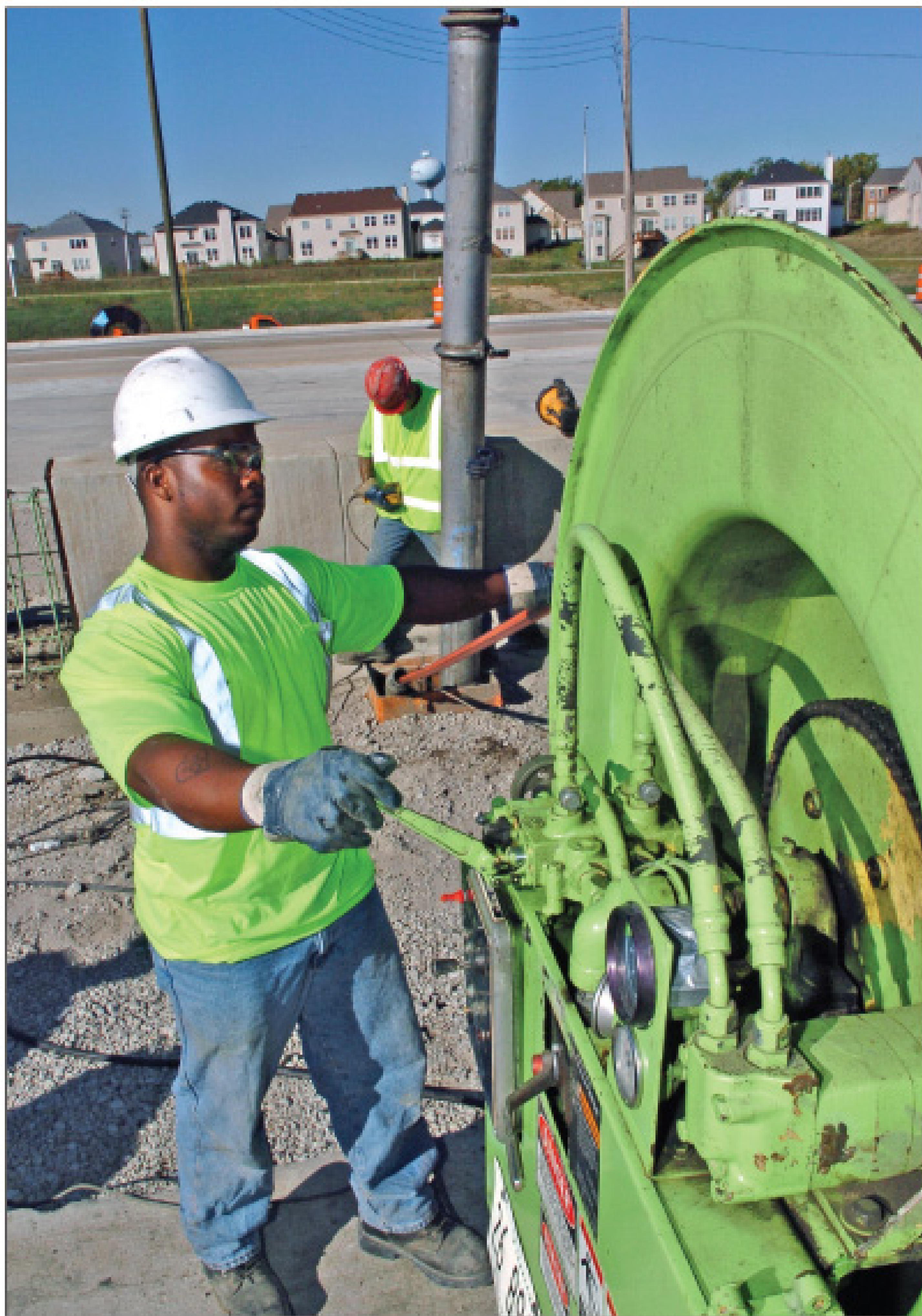
Larry Jeffries operates the jetter on a combination unit as Chuck Cushing vacuums debris.
