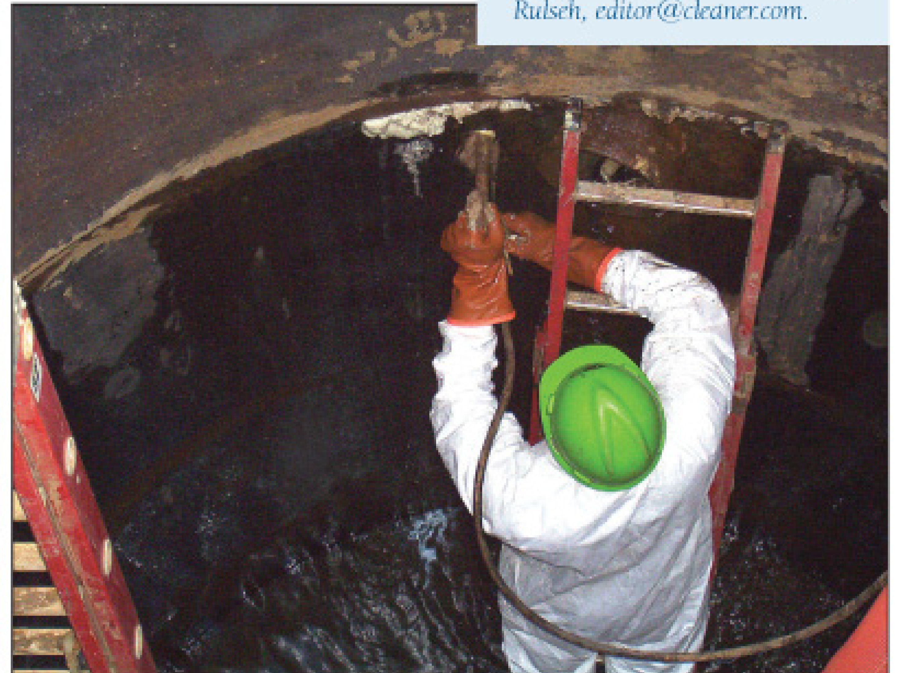
An injection specialist uses chemical grout to repair a leaking joint.
