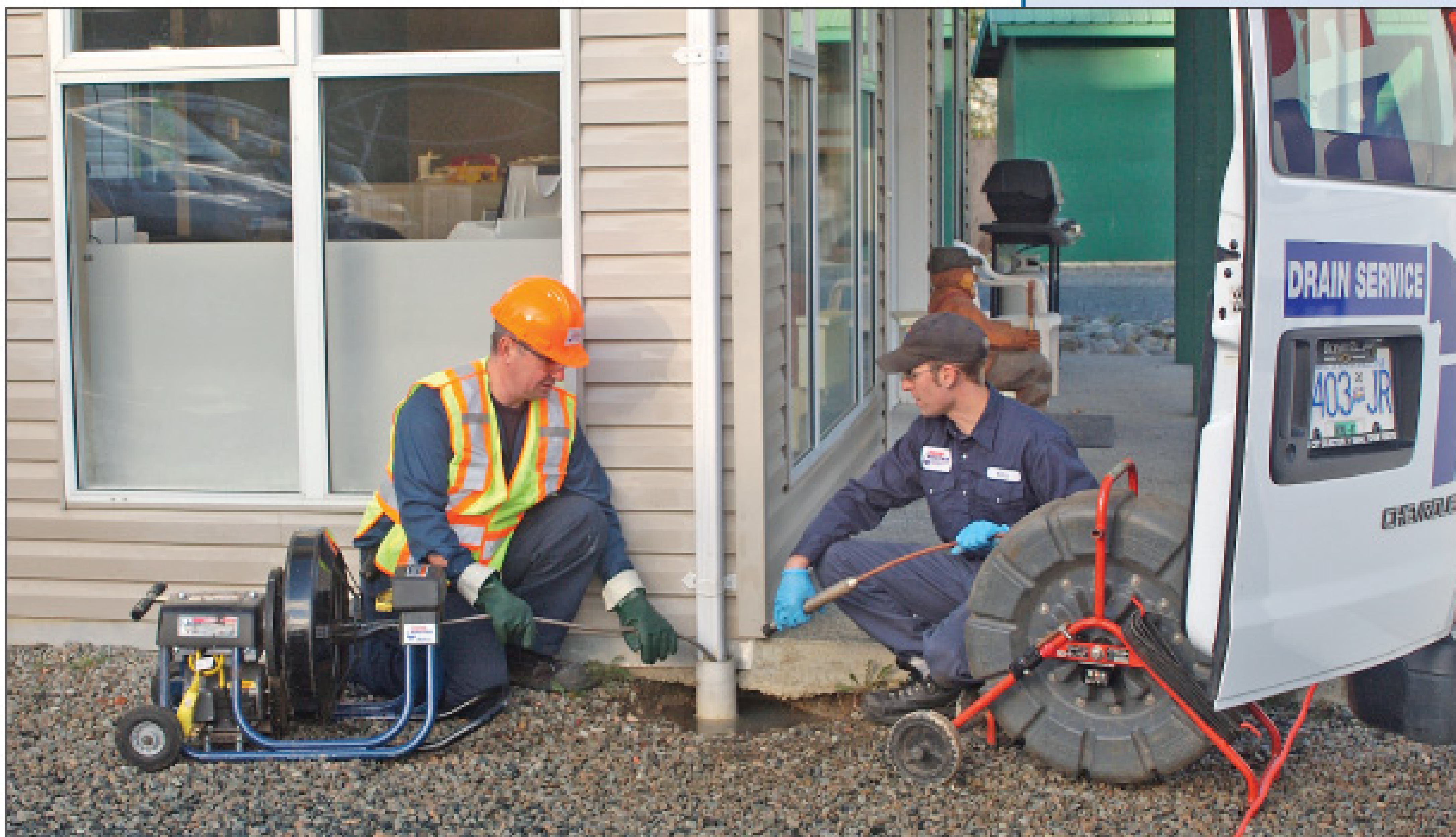
Technicians Travis Young and Kris Bergen auger a downspout.
