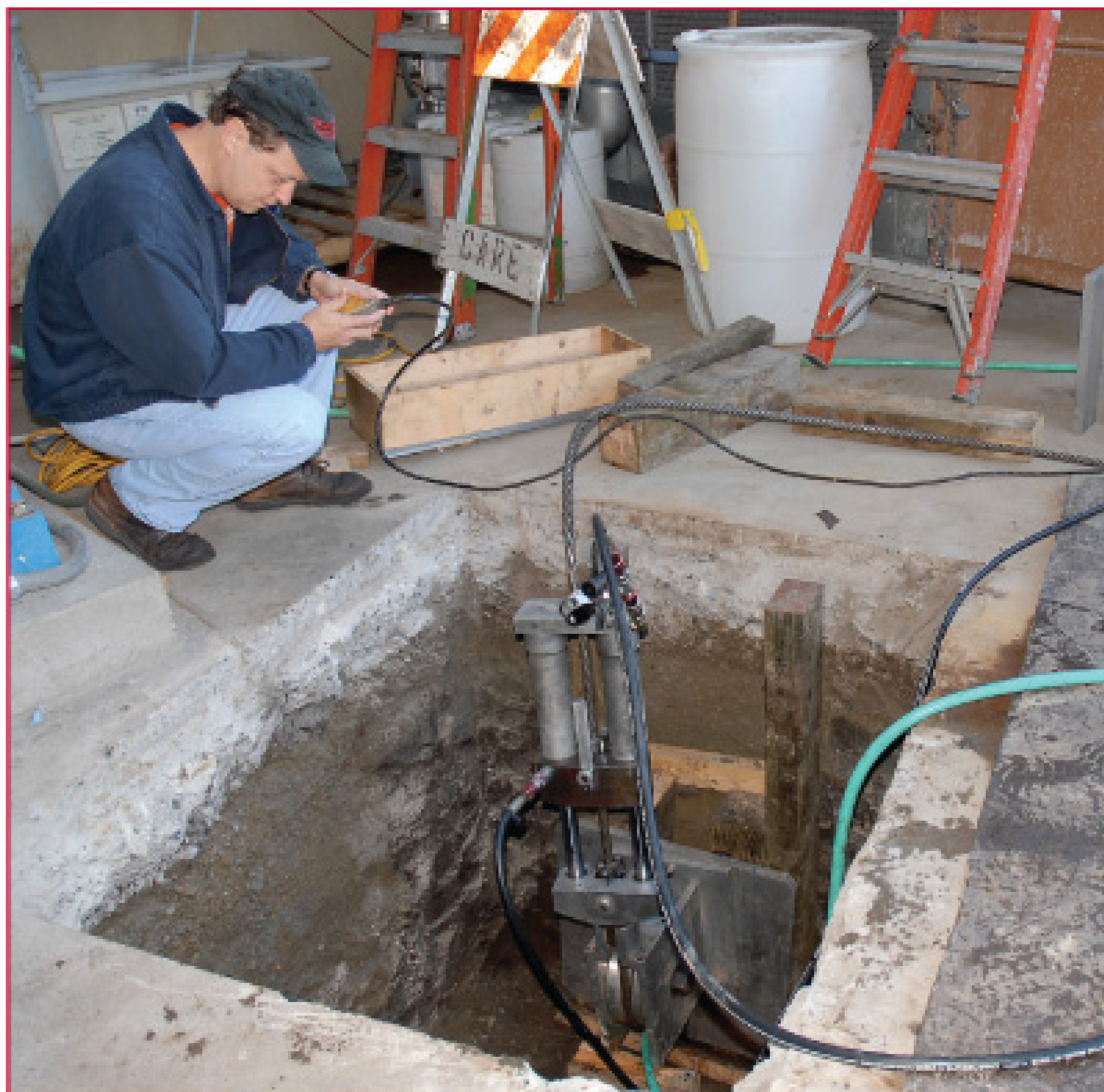
Michael Lien of TRIC Tools keeps an eye on the puller's pressure gauge.
