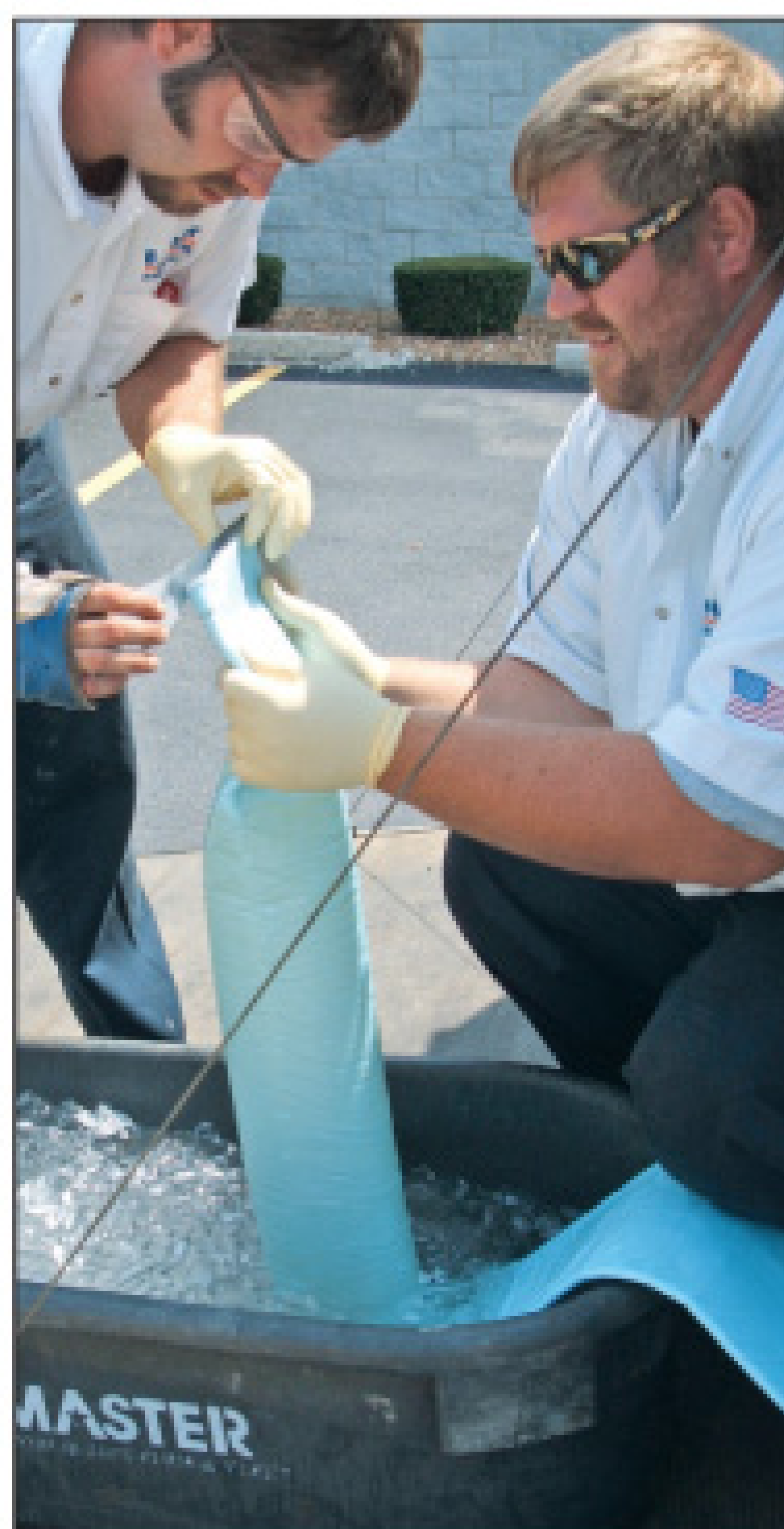
Technicians Bill Forrest and Mike Kampenga seal the end of the liner. An ice trough is used to cool the liner once the resin has been introduced.
