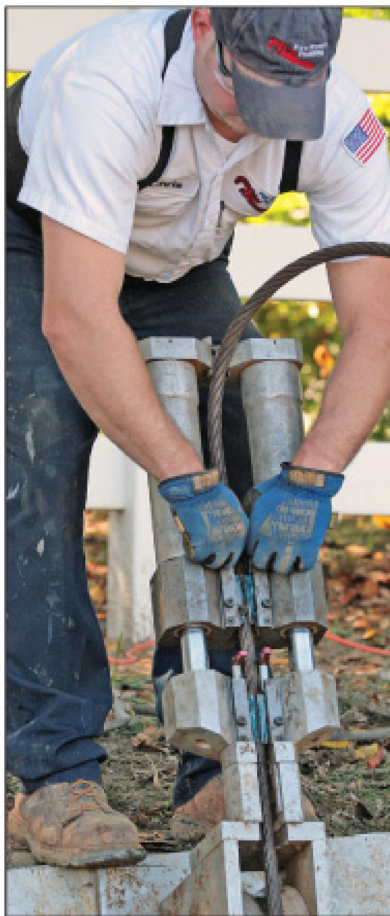
Technician Chris Phillips prepares for a pipe bursting job.
