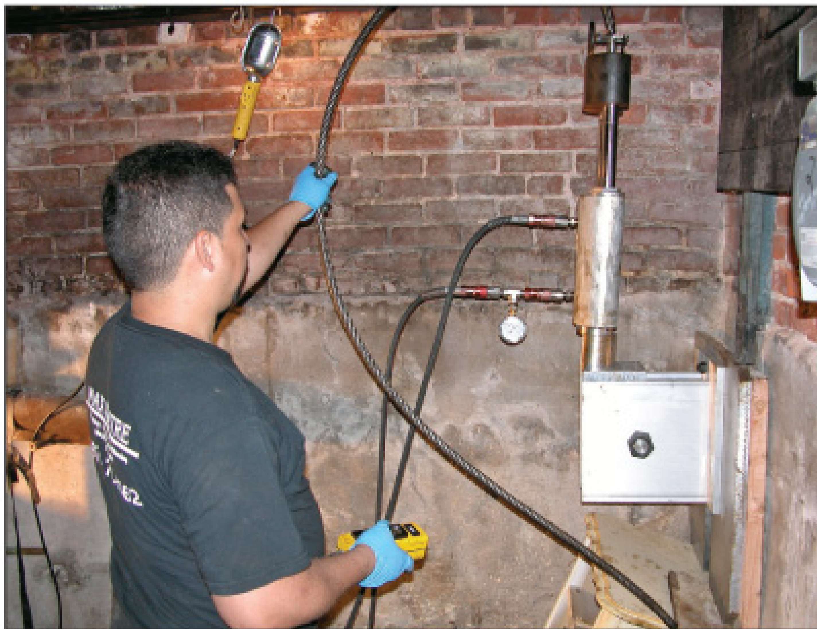
A static lateral bursting system pulls a 4-inch sewer into a basement.
