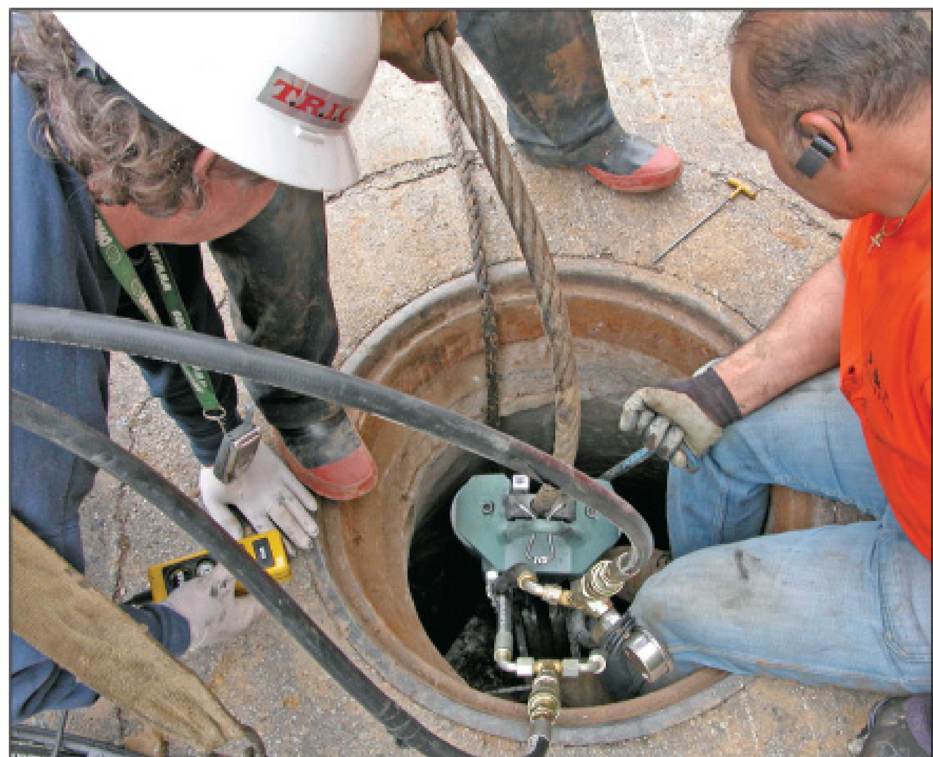
A 60-ton static puller uses 1-inch cable to burst an 8-inch clay sewer main. (Photos courtesy of TRIC Tools Inc.)
