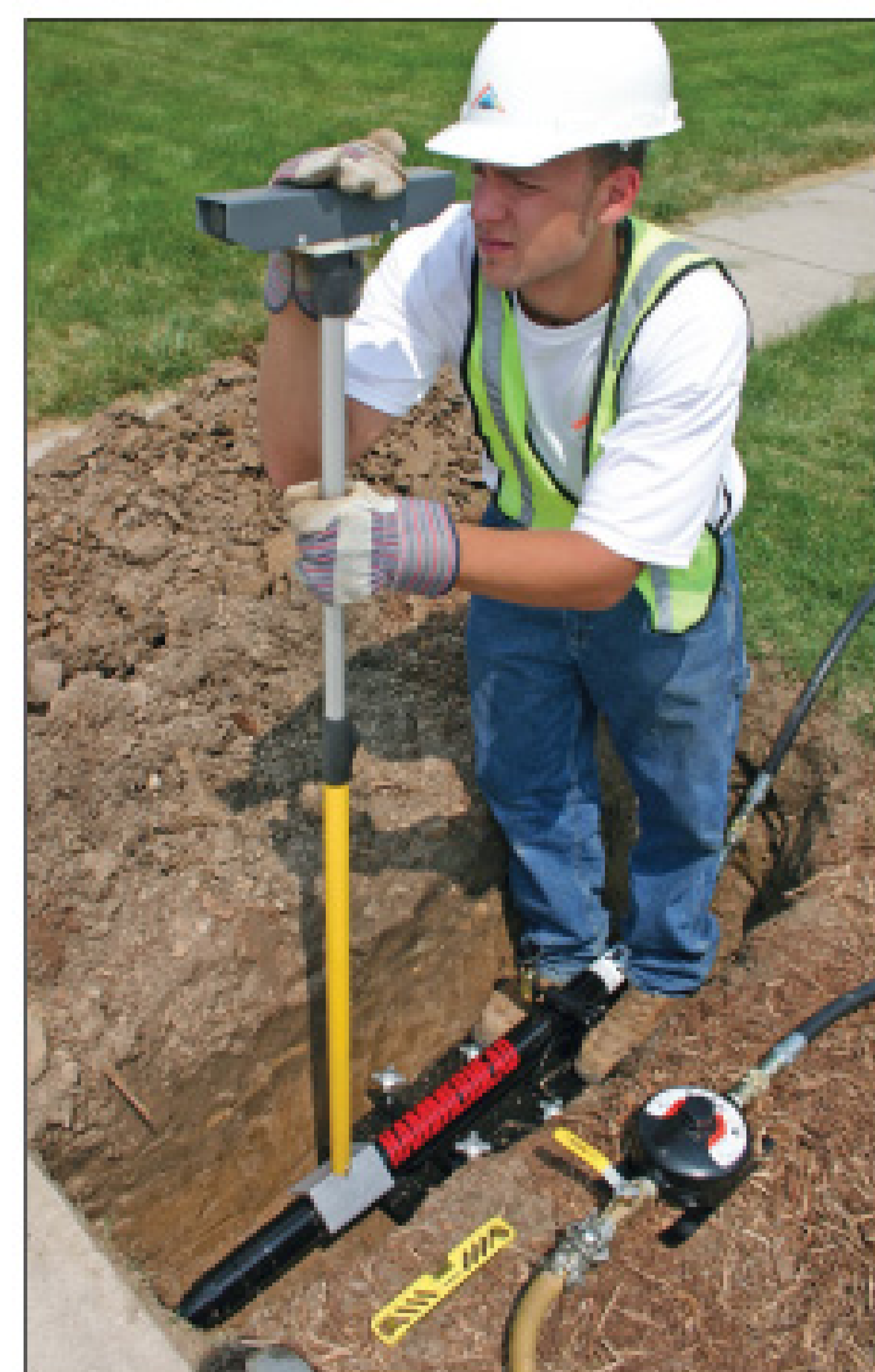
HammerHead Mole piercing tools from Earth Tool Company LLC
